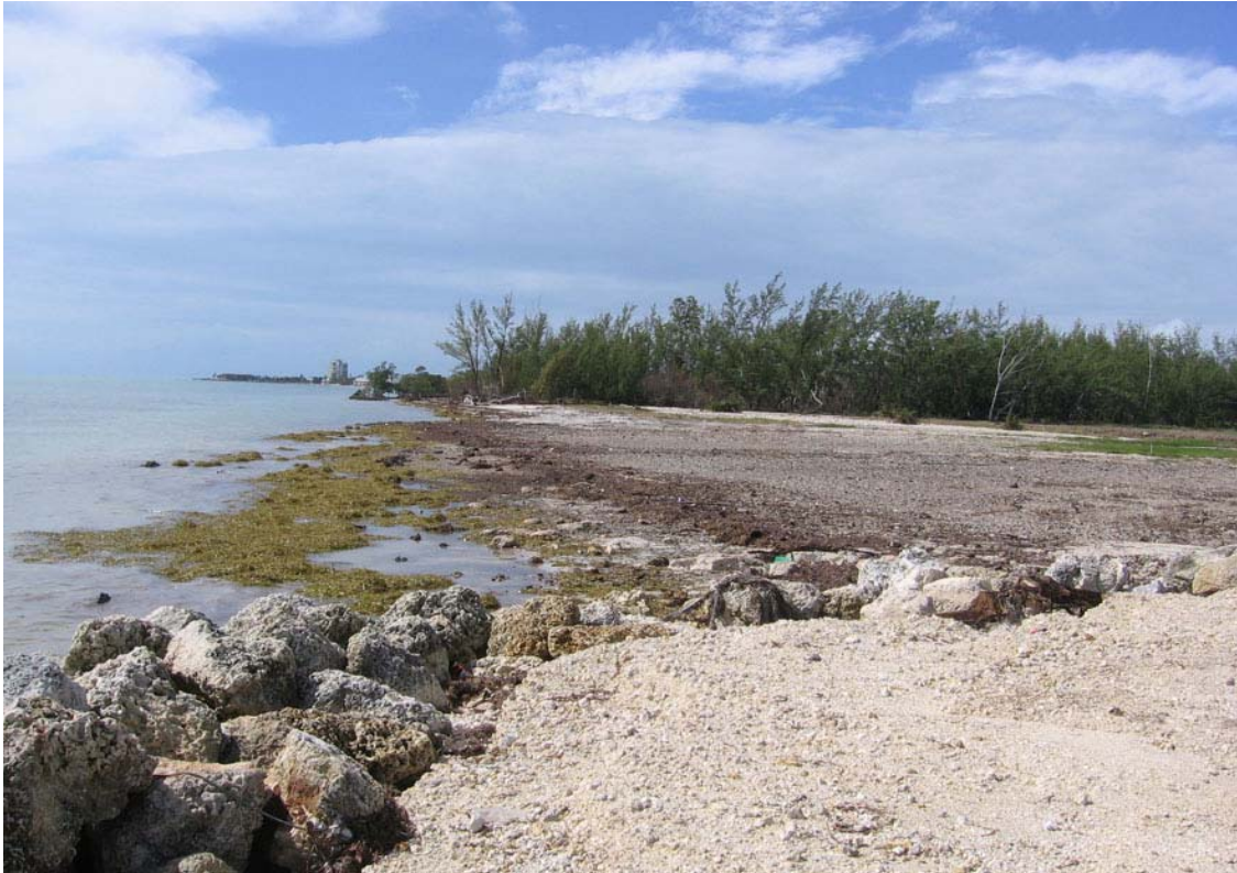
Photo 19. Severe beach erosion, Coco Plum beach.
