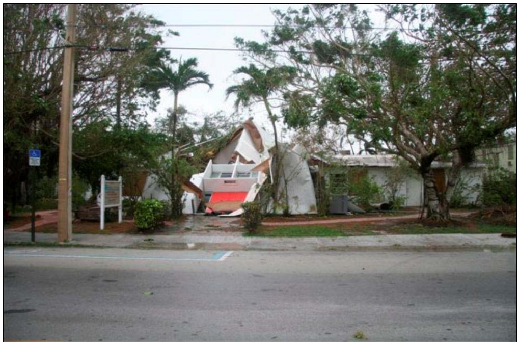
Photo 54. Key West wind damage.
