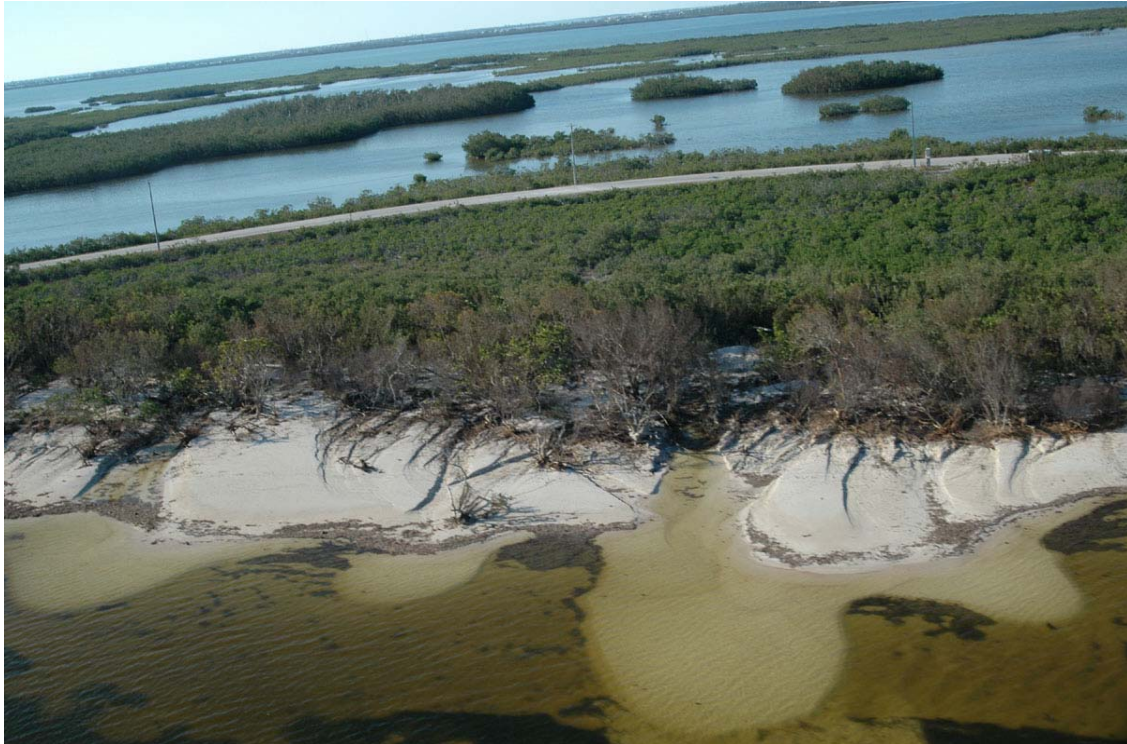
Photo 26. Storm surge discharge channels, Long Beach, Big Pine Key.
