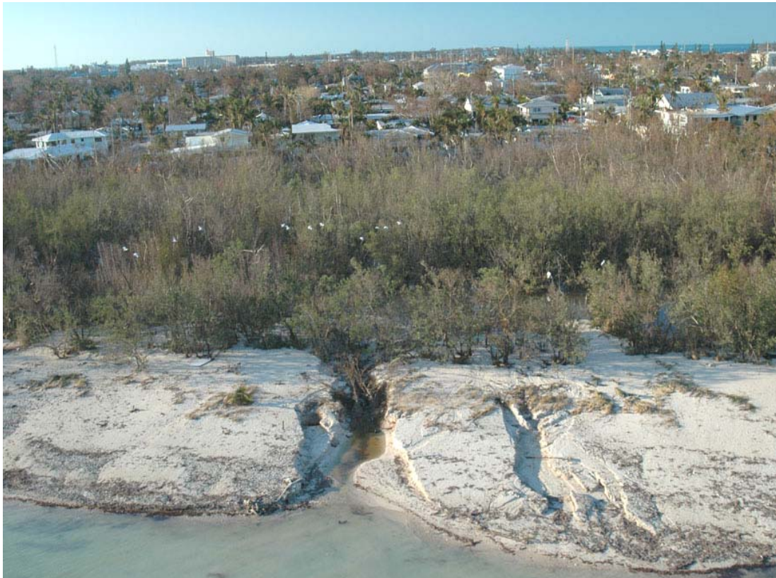
Photo 30. Scour channel, Berg and Kitsos Beach.
