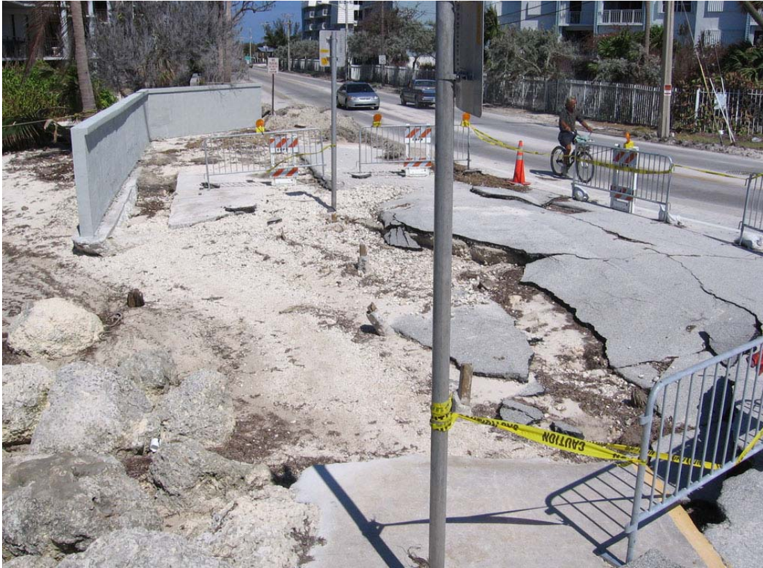
Photo 41. Pavement damage by Rita at Bertha Street, Key West.
