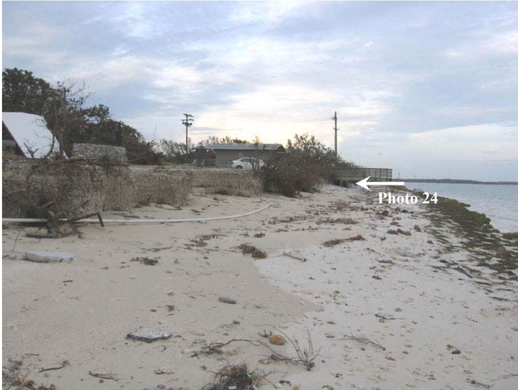
Photo 23. Severe erosion at Loggerhead Beach, Bahia Honda State Park.
