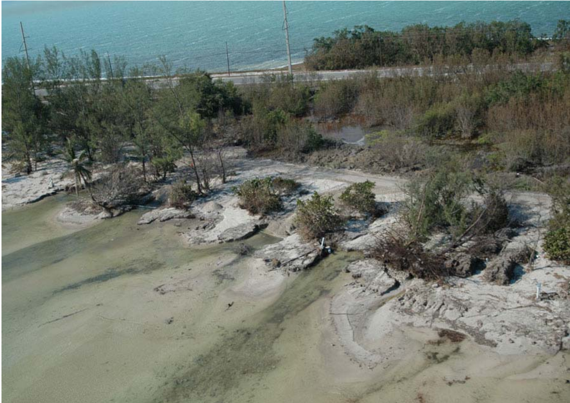
Photo 17. Storm surge scour channels, Long Key State Park.
