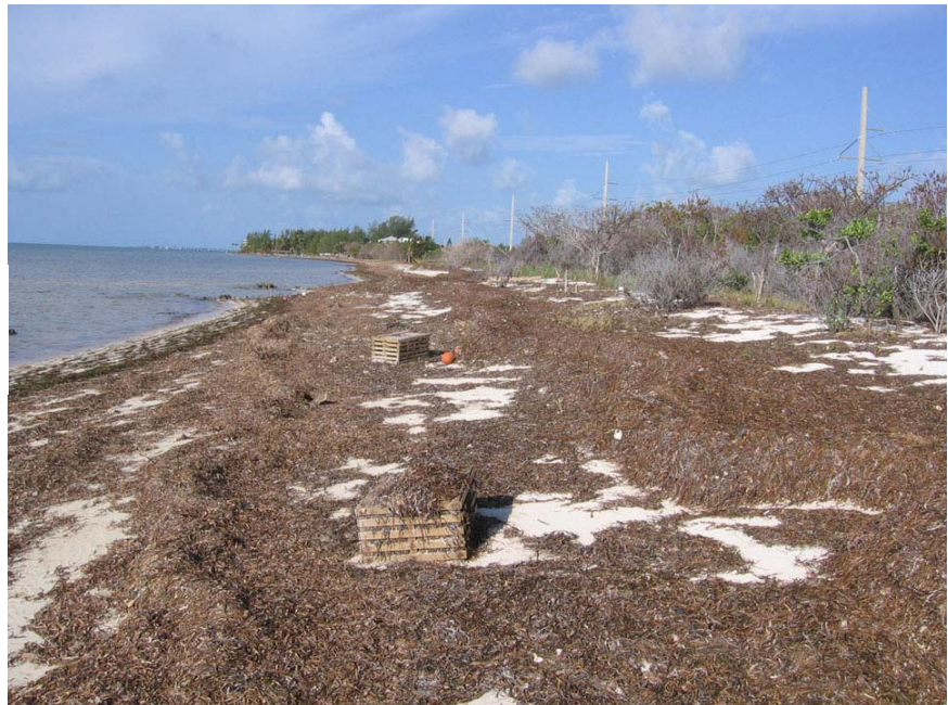
Photo 7. Beach erosion at Long Key State Park.
