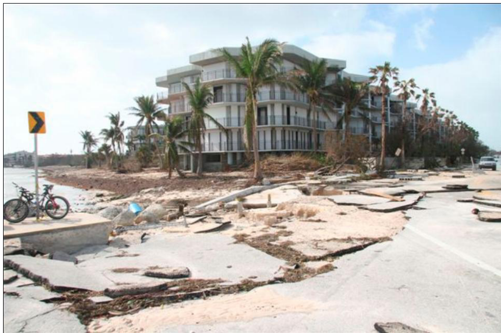
Photo 56. Bertha Street damaged (credit: City of Key West).
