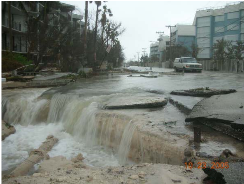
Photo 55. Bertha Street during Wilma's falling storm surge (credit: City of Key West).
