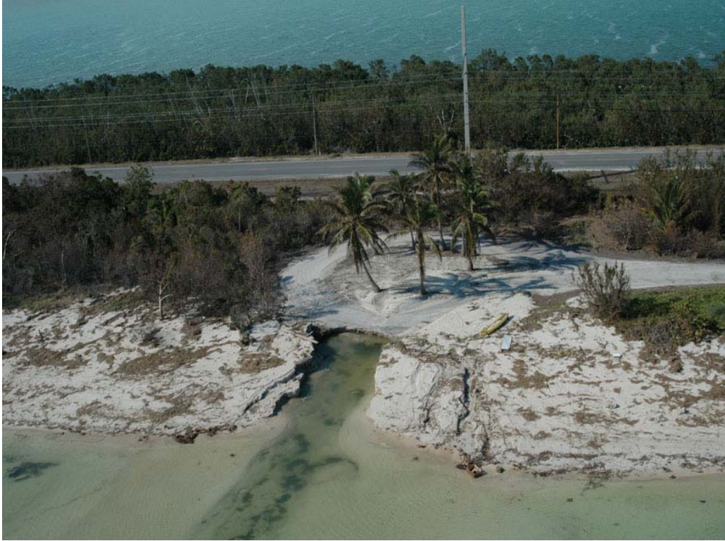
Photo 42. Storm surge discharge gully, Long Key State Park (Hurricane Wilma).
