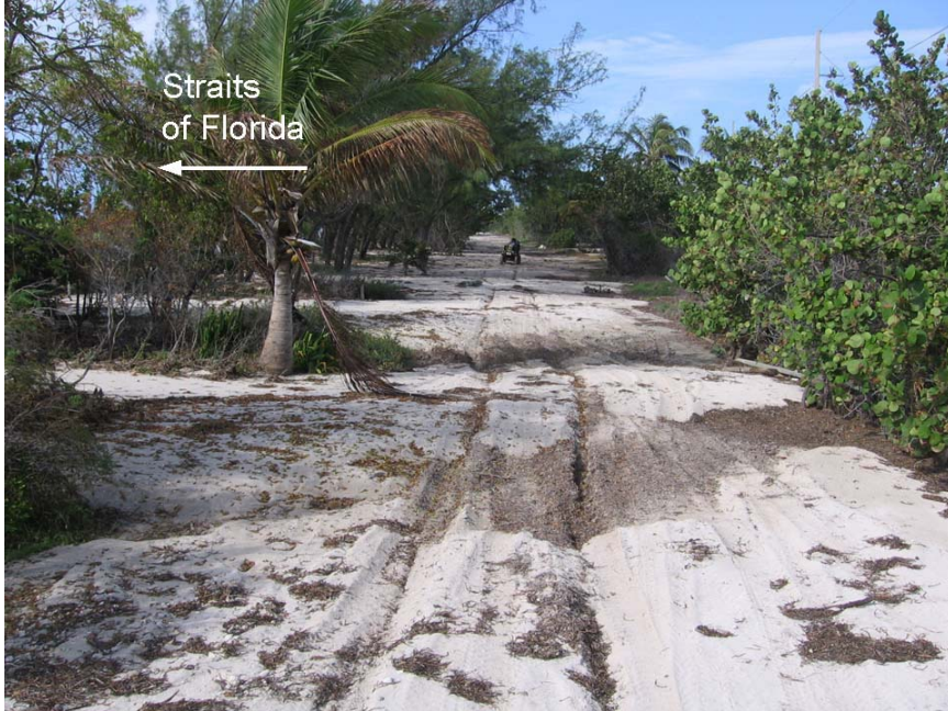
Photo 6. Overwash at Long Key State Park.
