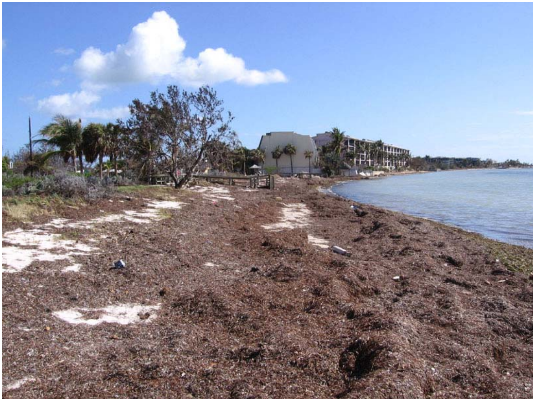
Photo 11. Minor beach and dune erosion at Rest Beach, Key West.
