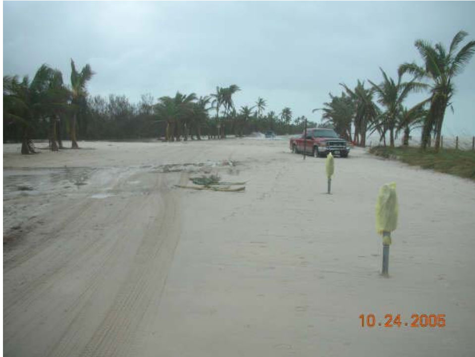
Photo 28. Overwash from Smathers Beach onto South Roosevelt Boulevard (credit: City of Key West).
