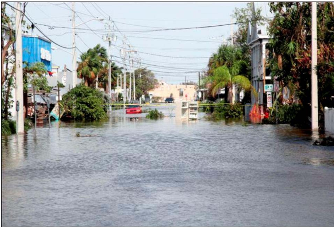
Photo 14. Key West flooding (credit: City of Key West)
