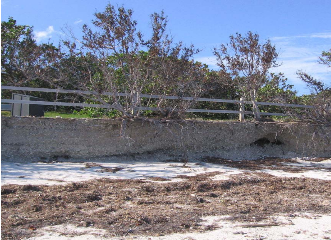
Photo 10. Moderate beach and dune erosion at Loggerhead Beach.
