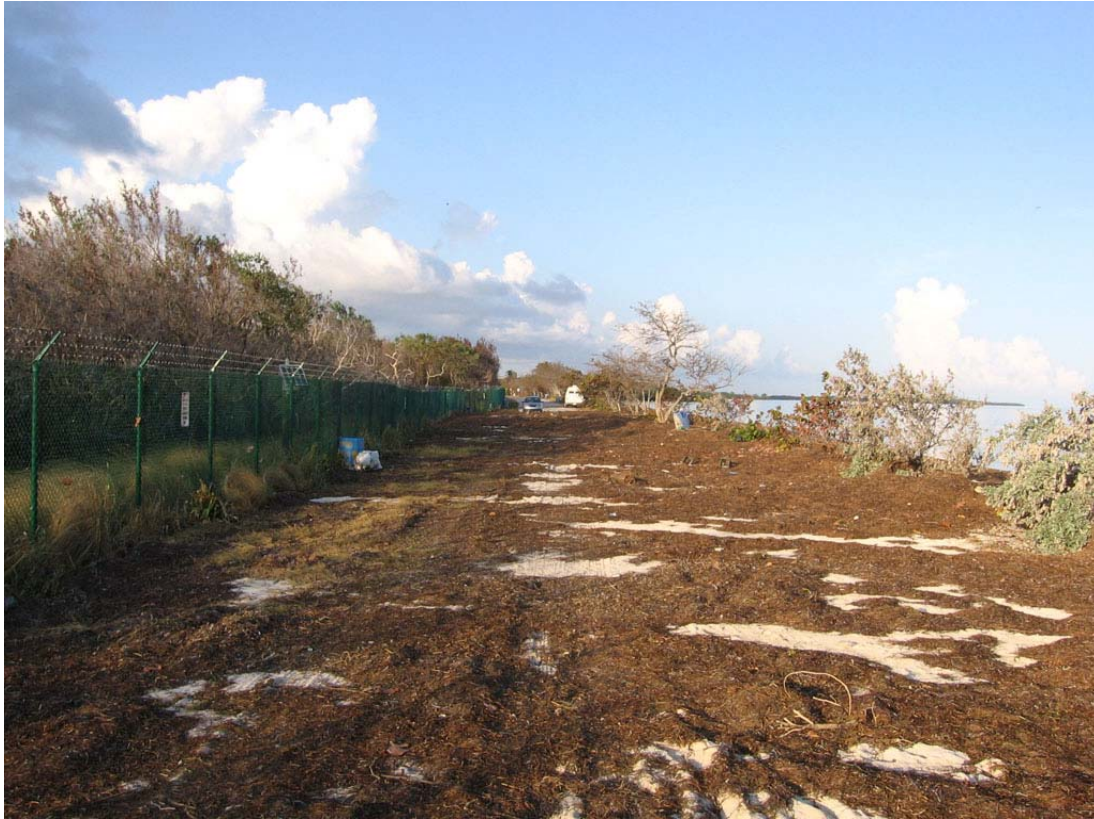
Photo 40. Roadway overwash by Rita at Boca Chica Beach.
