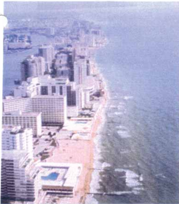
BEFORE PROJECT CONSTRUCTION
