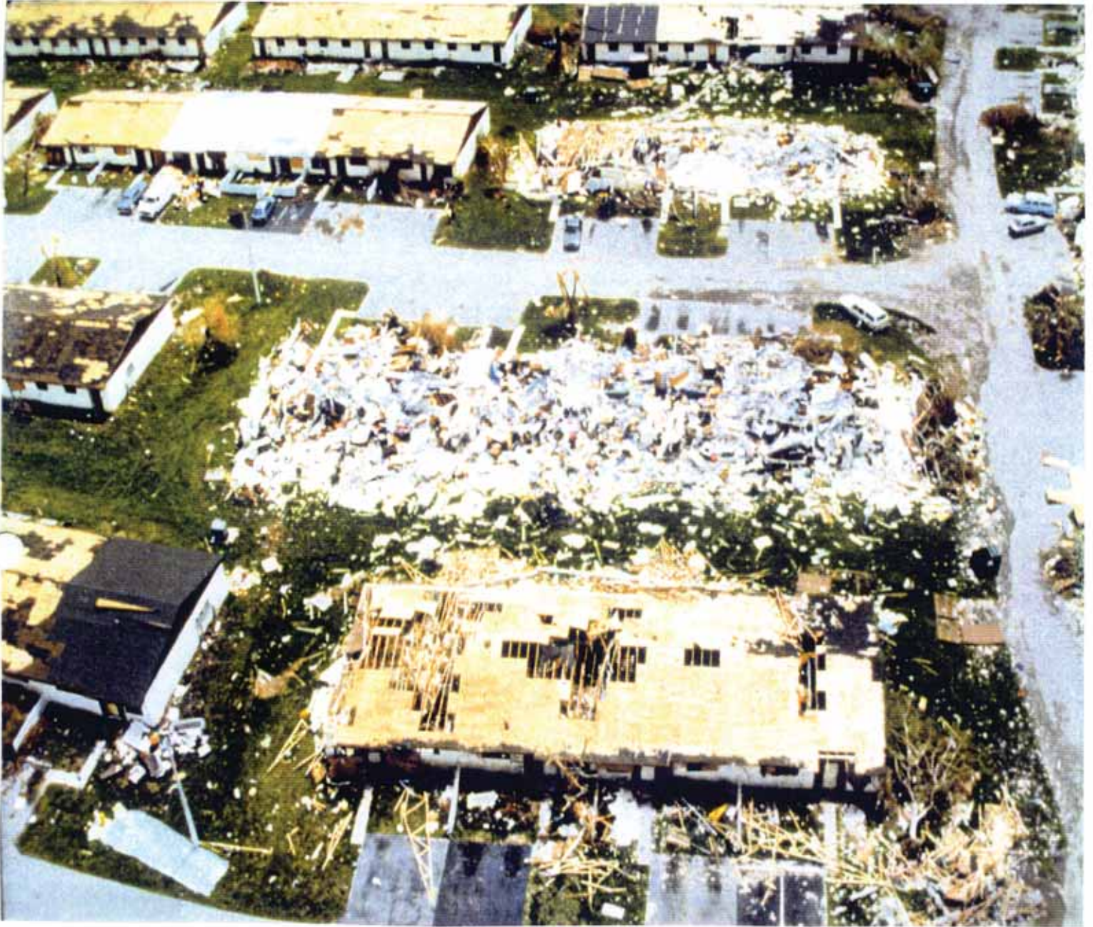
FIGURE 18 DAMAGE TO DUPLEX
