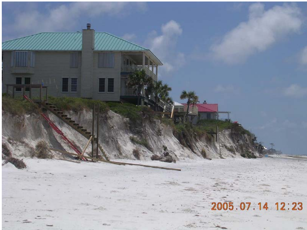
Photo 40. Imminently threatened structure, St. Joseph Peninsula (R91).
