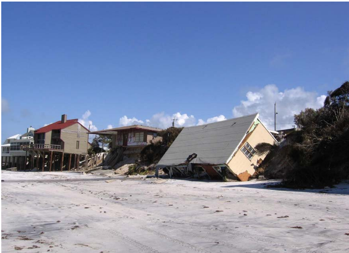
Photo 27. Dwelling destroyed, Inlet Beach (R123).
