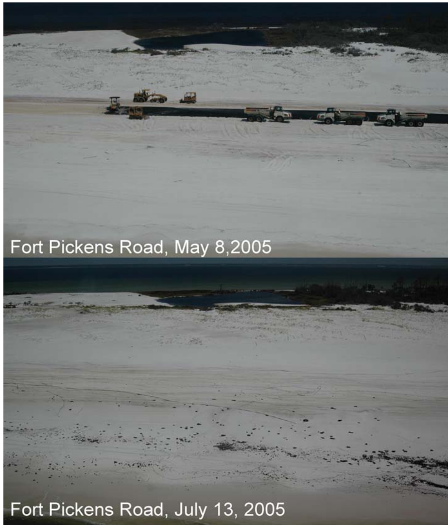
Photo 1. Fort Pickens Road before and after Hurricane Dennis.
