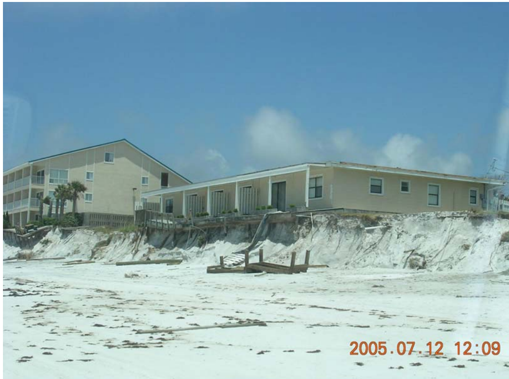
Photo 19. Multifamily dwelling undermined, Destin (R44.5).
