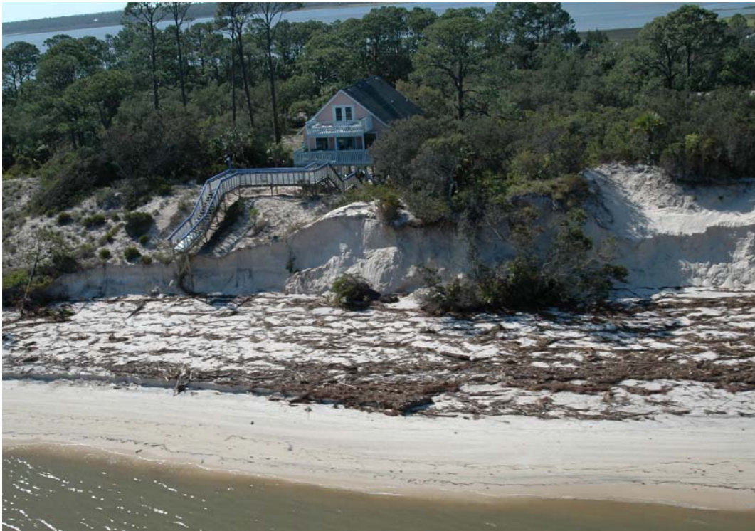
Photo 43. Dune erosion at Indian Pass (R160.4).
