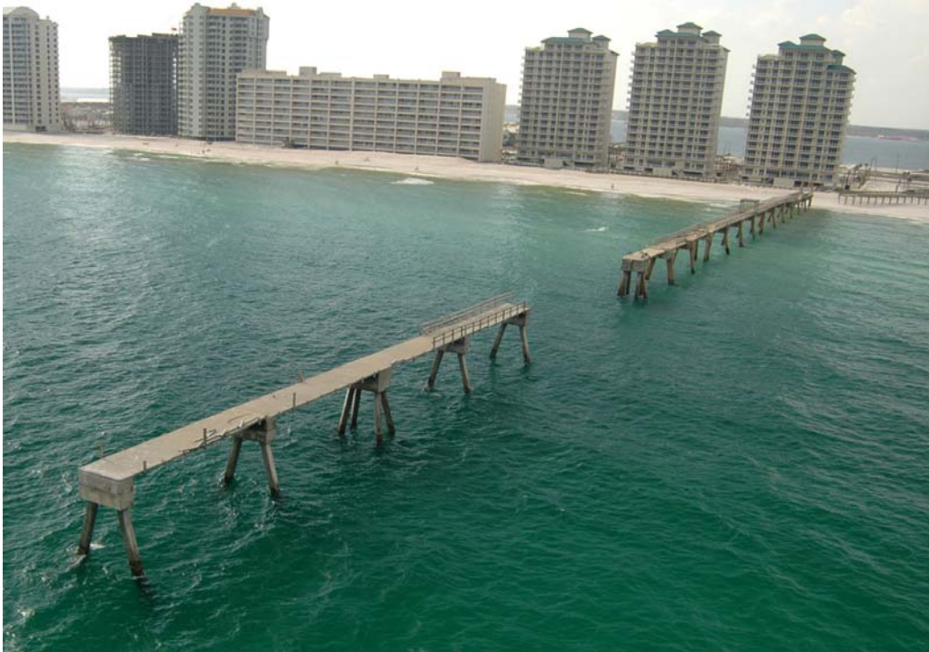
Photo 9. Damage to Navarre Fishing Pier (R209).
