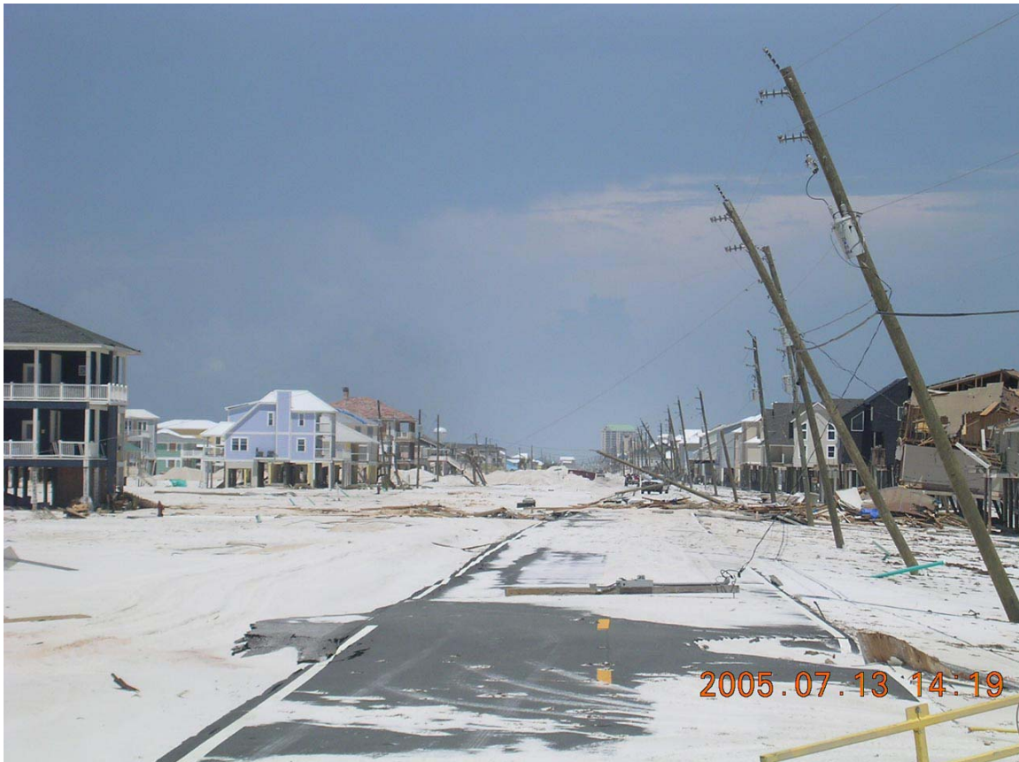
Photo 8. Infrastructure damage along Gulf Boulevard, Navarre Beach (R192.5).
