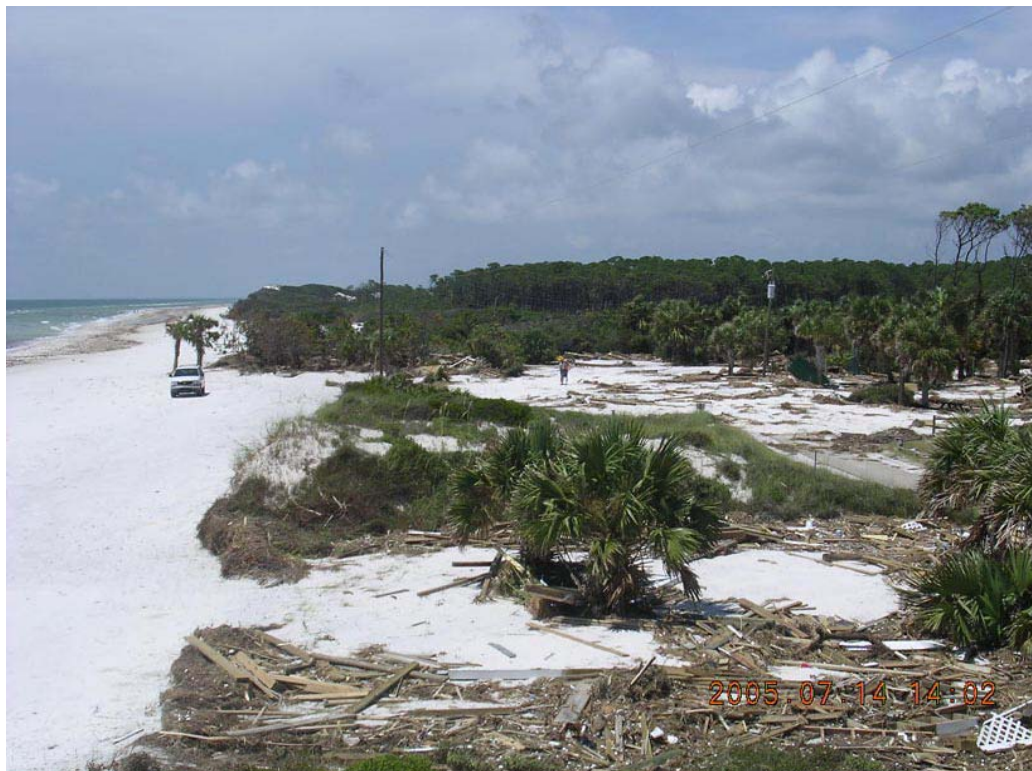
Photo 39. Dune breach at St. Joseph Peninsula State Park (R69).
