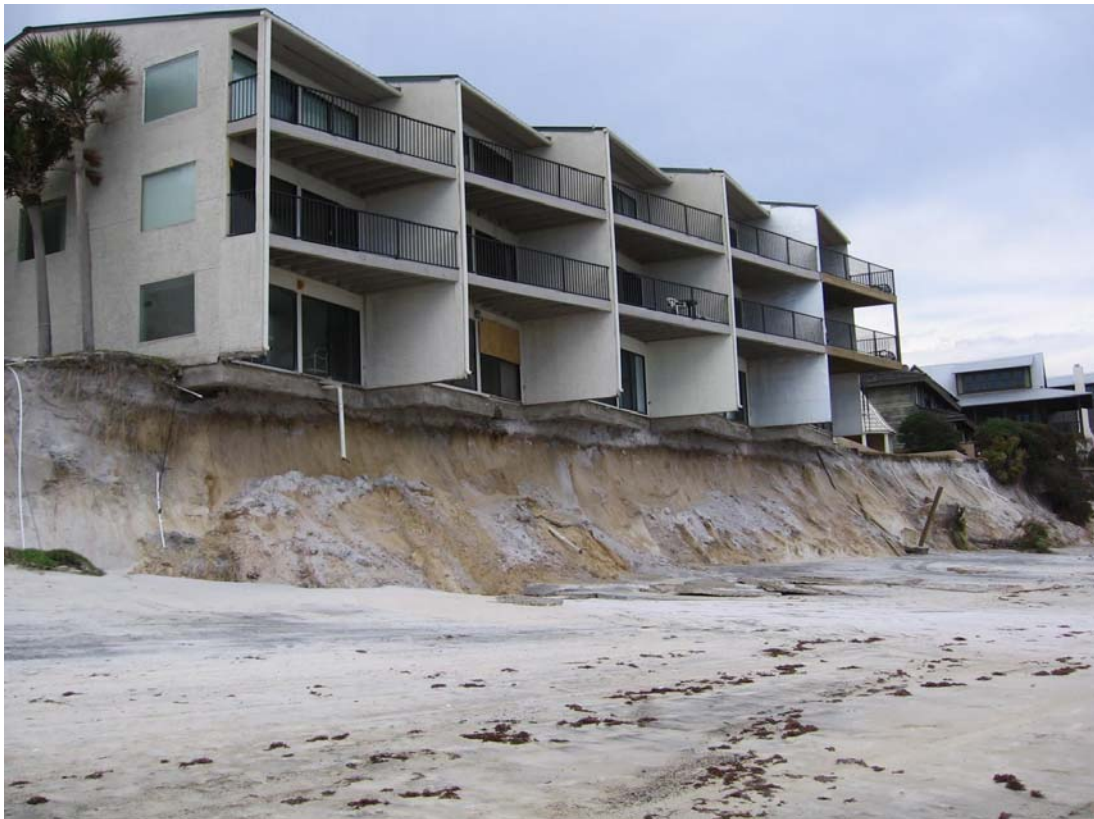
Photo 24. Imminently threatened building, Blue Mountain Beach (R60).
