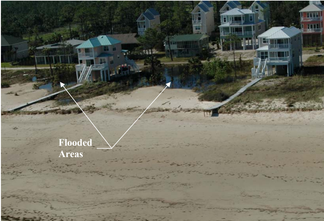
Photo 42. Significant flooding near Money Bayou (R141.5).
