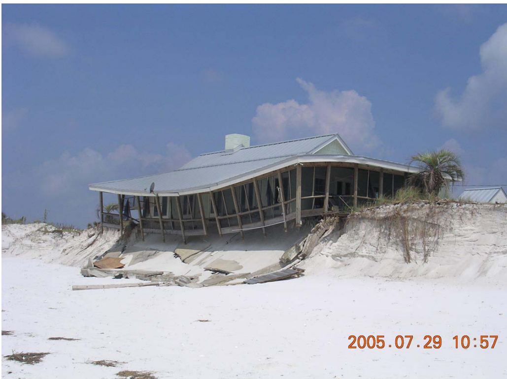
Photo 55. Dwelling undermined and damaged, Dog Island (R176.2).
