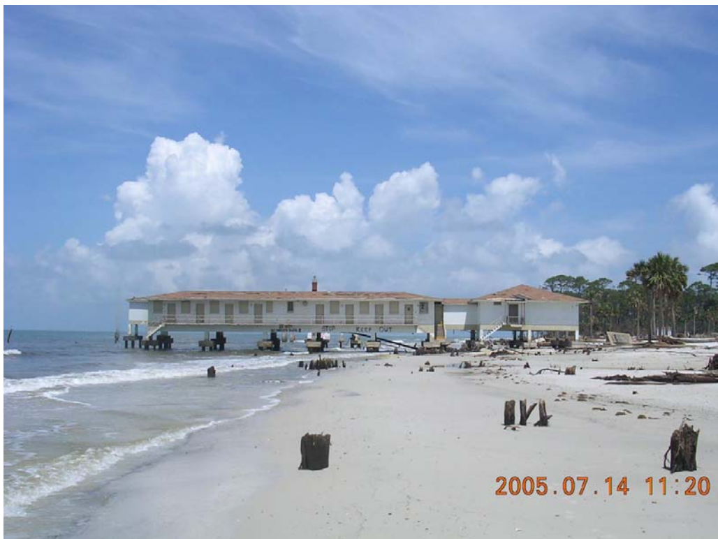
Photo 41. Severe beach erosion at the Cape San Blas Lighthouse (R111.5). (Structure depicted in photo has been removed.)
