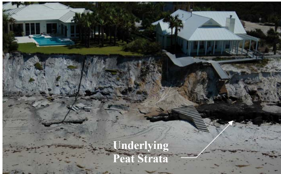
Photo 26. Imminently threatened structure, Seacrest Beach (R112.4).
