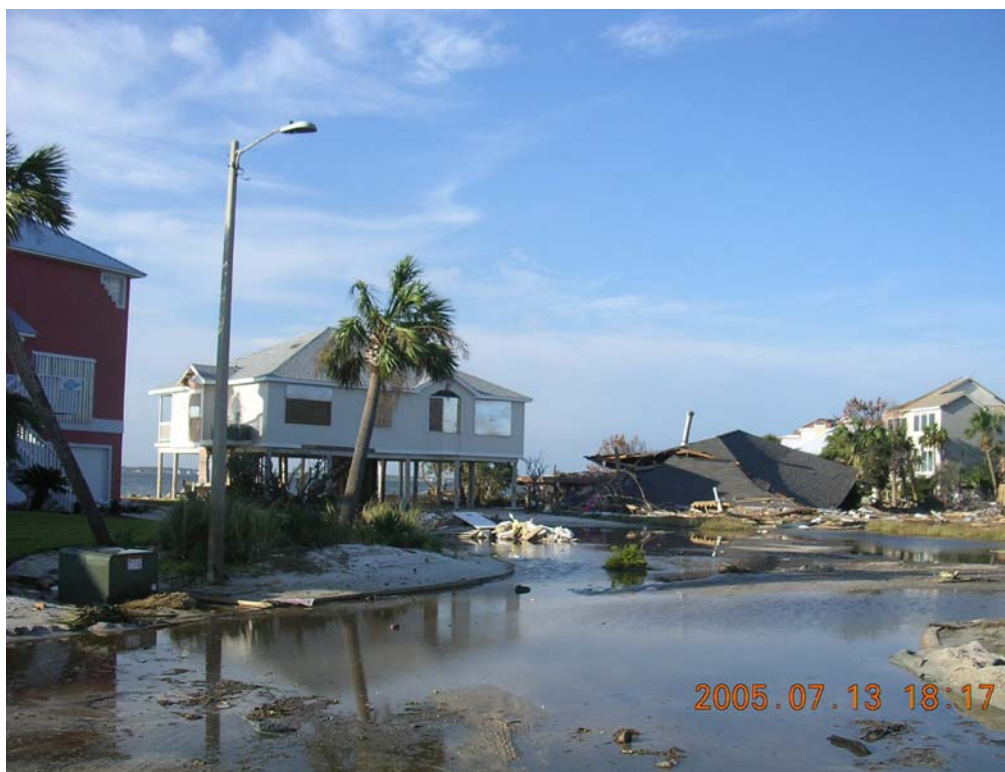
Photo 2. Destroyed dwelling, Pensacola Beach.
