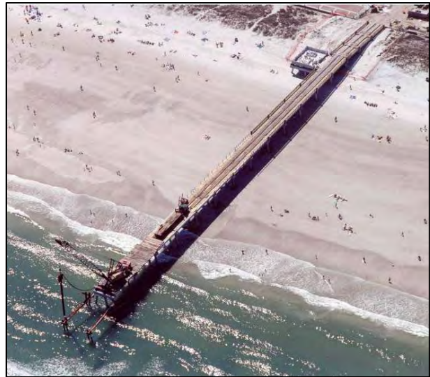
Figure 14: Pier under construction. Source: PBS&J
