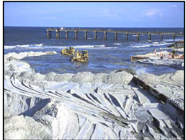
Sand Dike being constructed during beach nourishment. Source: PBS&J
