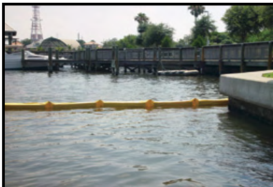
Use of a turbidity barrier for a small-scale project. Source: http://www.dawginc.com/secondary-spill-containment/turbidity-barrier-curtain.php
