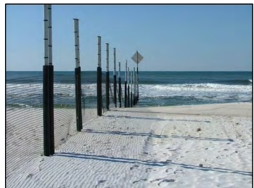
Figure 16: Net groins at Eglin Air Force Base. Source: PBS&J
