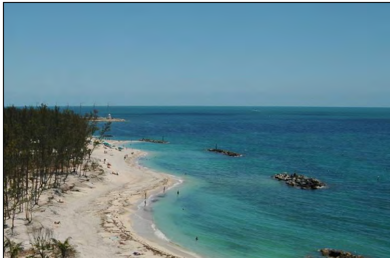
Figure 13: Sub-aerial breakwaters, Key West. Source: PBS&J
