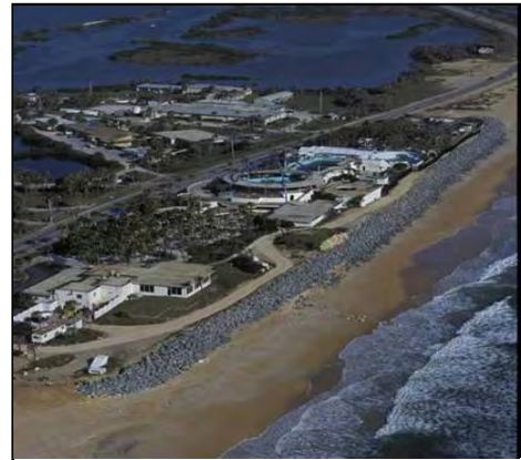
Figure 11: Revetment at Marineland. Source: PBS&J
