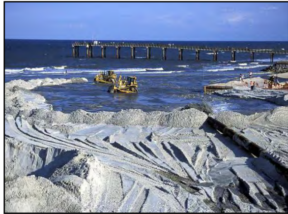
Figure 9: Sand dike construction.
