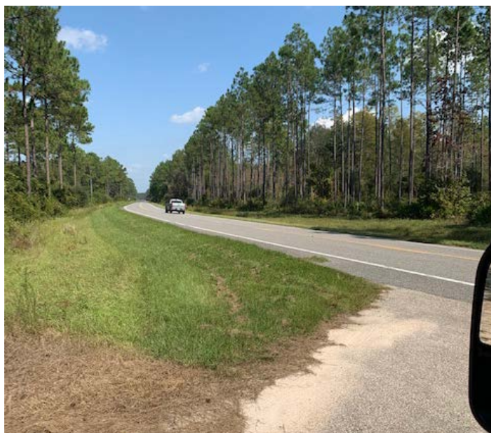
View of Gamble Rd/ SR 59 looking northeast
