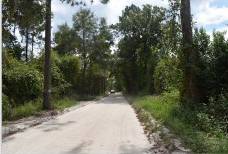
PHOTO #5 VIEW OF OLD SHELL POINT ROAD LOOKING SOUTH
