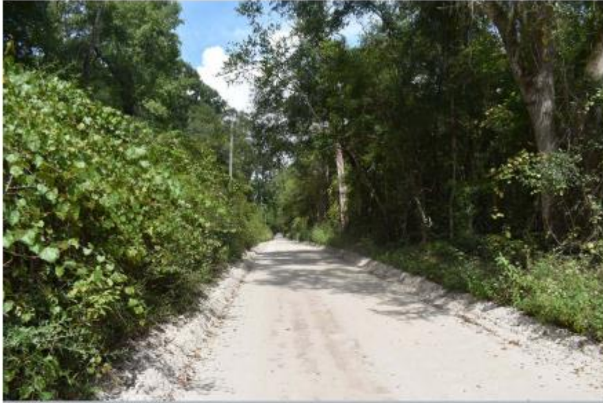
PHOTO #1 VIEW OF OLD SHELL POINT ROAD LOOKING NORTHEAST
