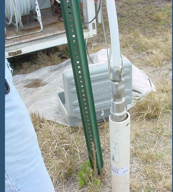
Submersible pump lowering into well.
