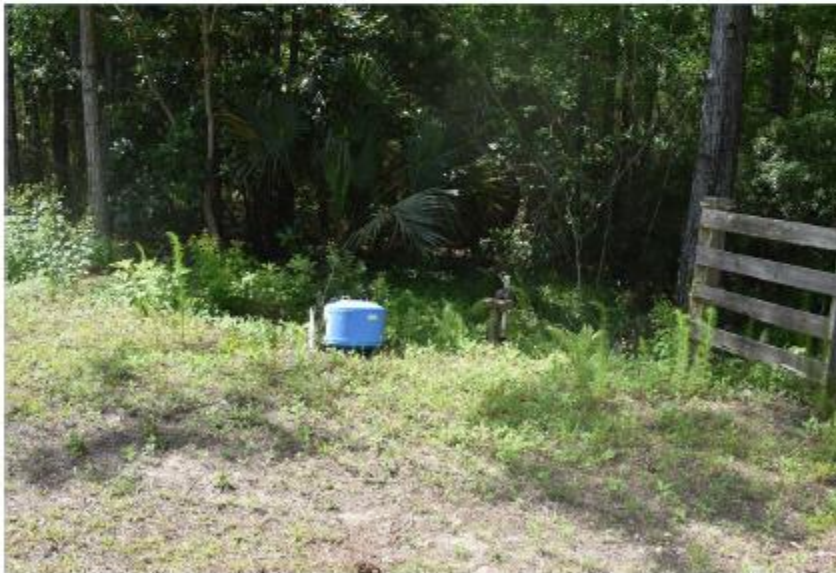
VIEW OF ONE OF FOUR TEST WELLS ON SITE CORDING TO BROKER, THE WATER WAS FOUND TO BE POTABLE
