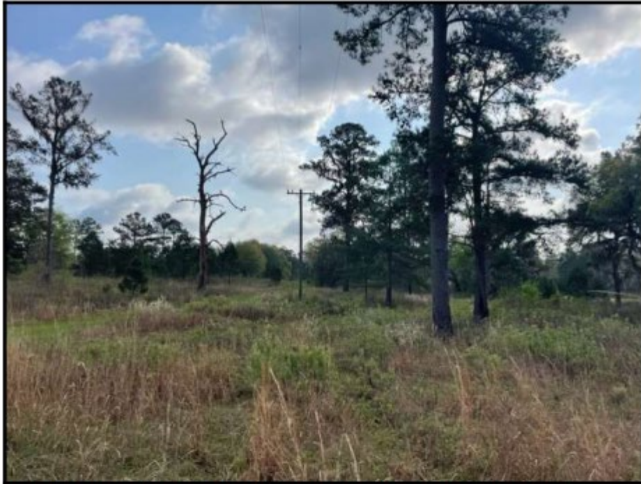
Photo7: Representative view of local electrical service line extending through the site.
