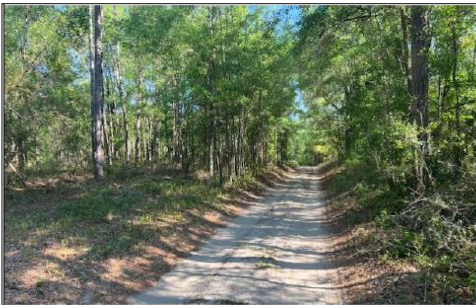
Subject- Interior Road
