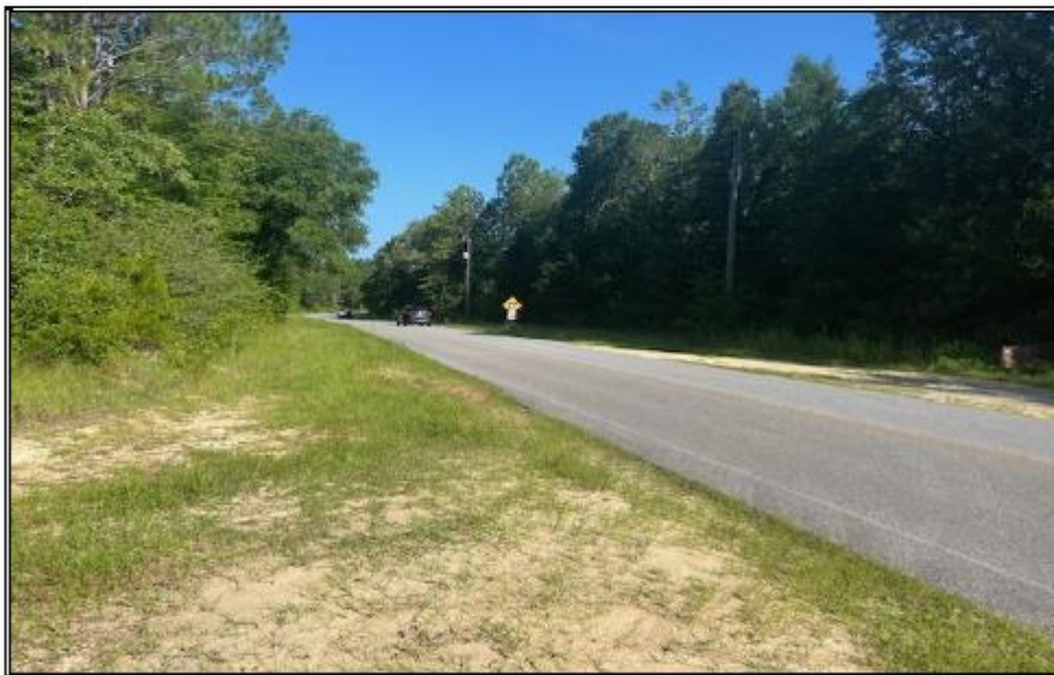
Street Scene- King Lake Road- Facing North
