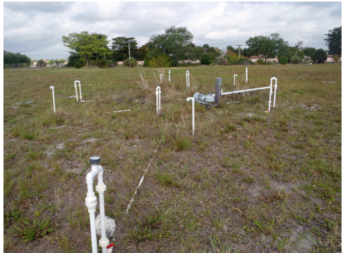
Above: Bio-sparge remediation system at the McArthur Dairy Brownfield Site
