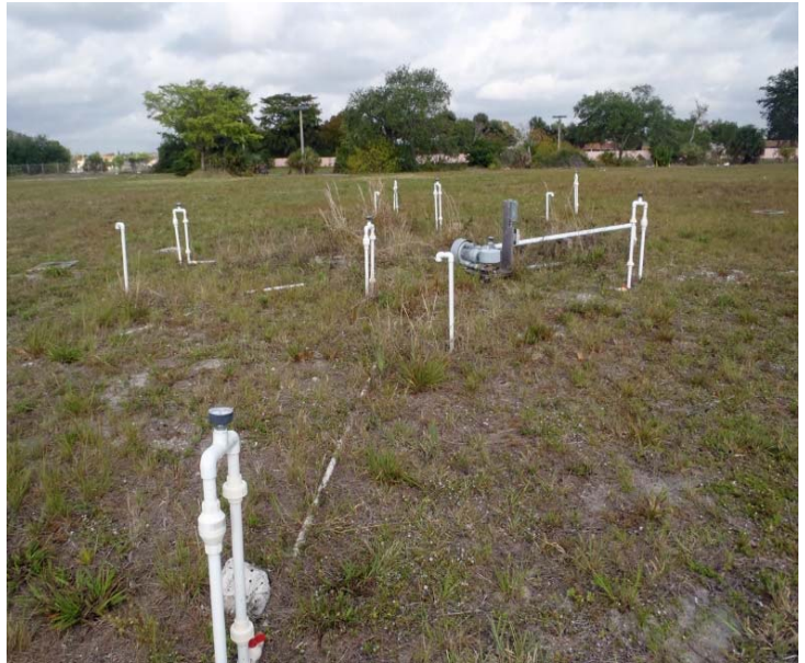
Above: Bio-sparge remediation system at the McArthur Dairy Brownfield Site
