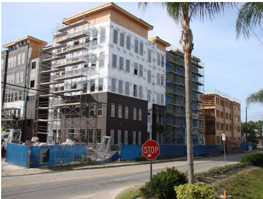
Spruce Street Apartment Complex and Parking Garage Construction
