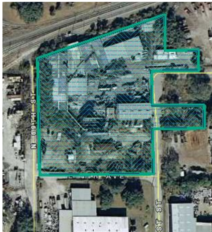
Gulf Coast Metals, aerial site view.
