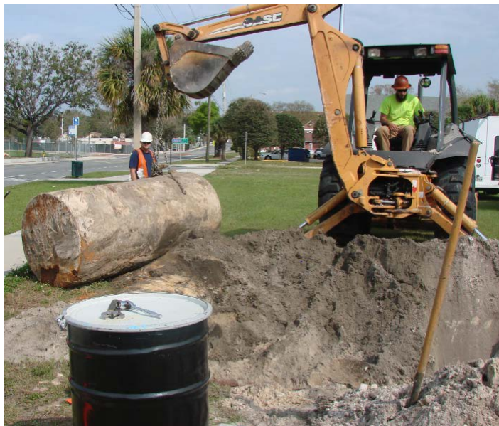
Small Tank Removal 2014
