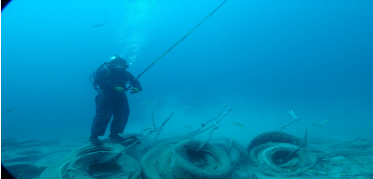
Figure 8. Surface air supplied diver hand bundling tires for transport to the surface by crane.
