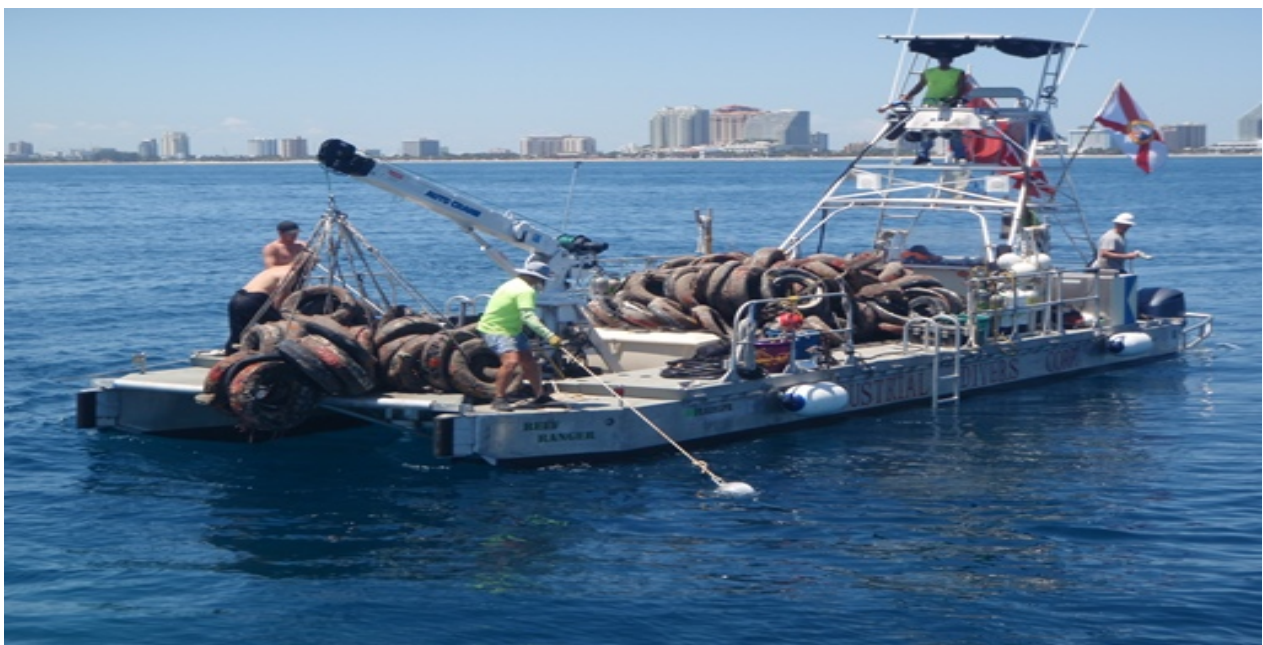
Figure 9. Current commercial tire removal operation using a similar method to that used by the military. Once the support vessel is loaded with approximately 500 tires, the vessel will return to Port Everglades to offload the tires into an open-top container.
