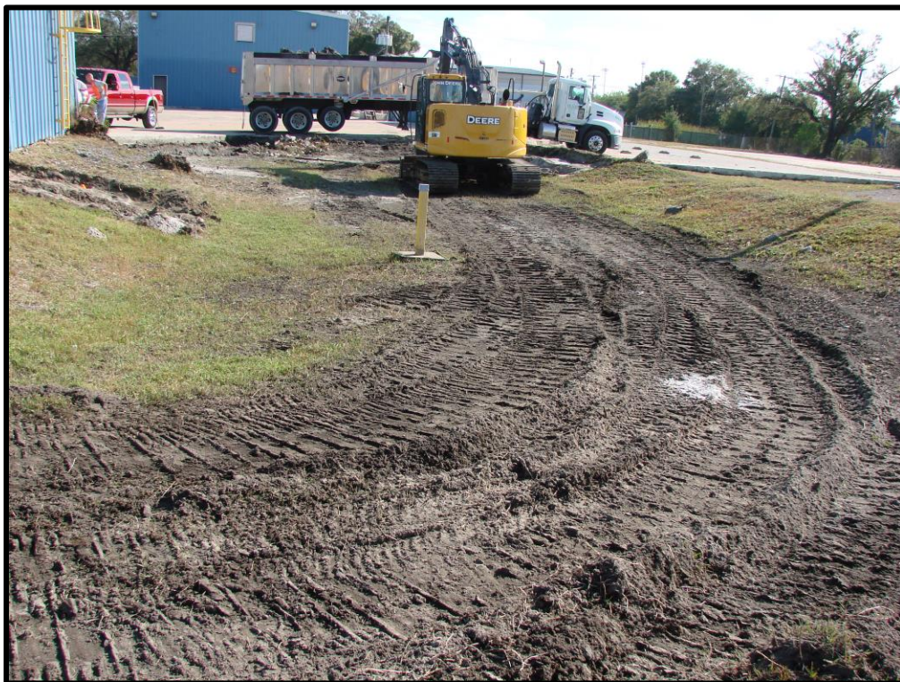
Soil Removal at the former Gulf Coast Metals site
