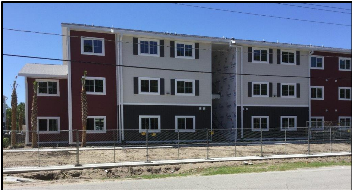
Sweetwater Villas under construction
