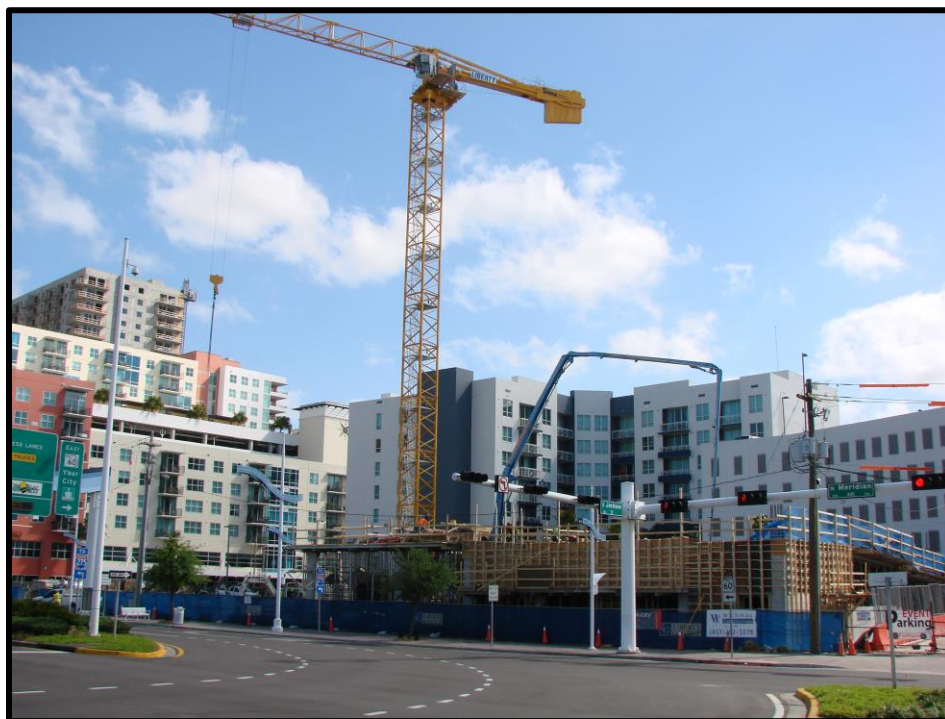
Liberty Tampa site under construction, March 2018
