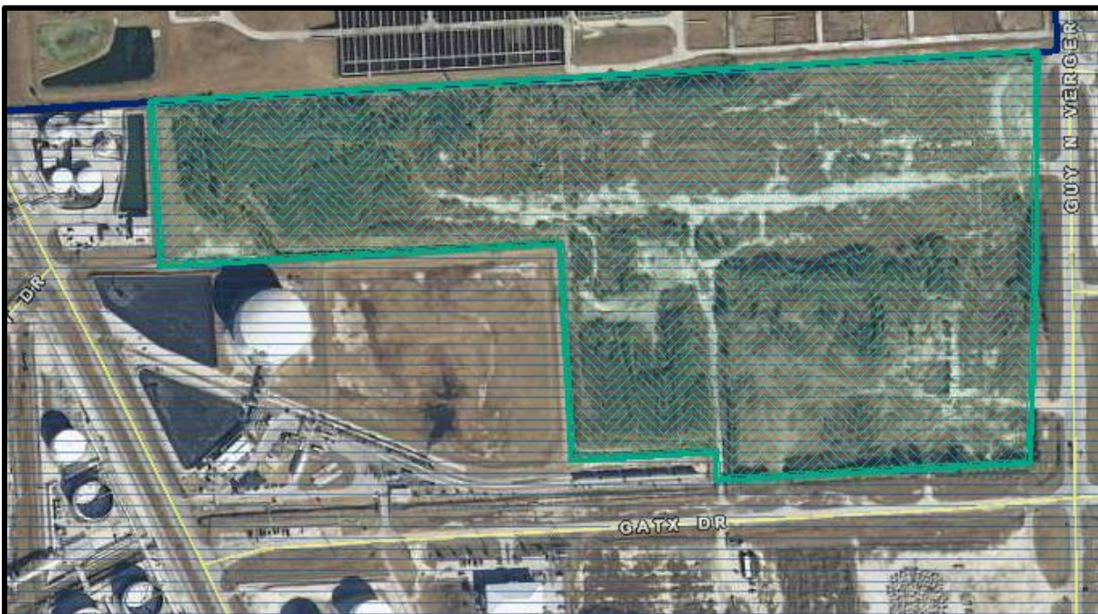
Aerial view of former Winner Metals site
