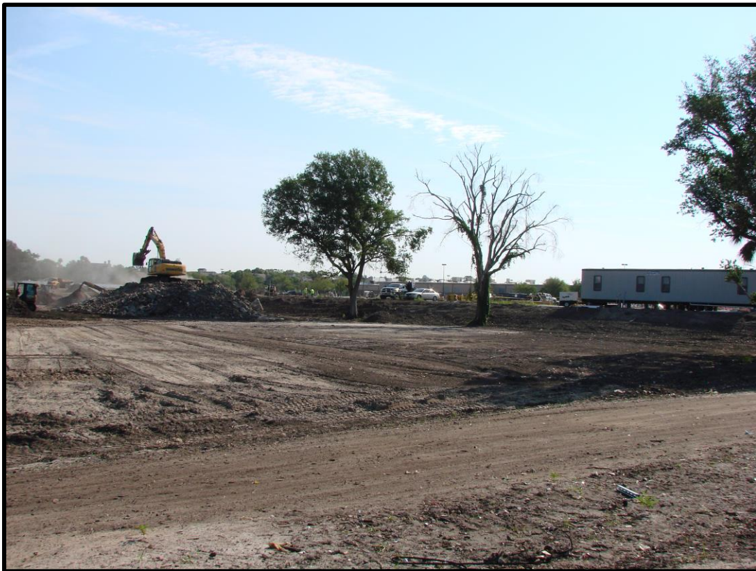
Grading at the Former Tampa Jai Alai Brownfield site
