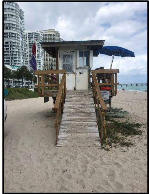
Lifeguard Tower 163 – 16301 Collins Avenue Adjacent to Beach Access 18
