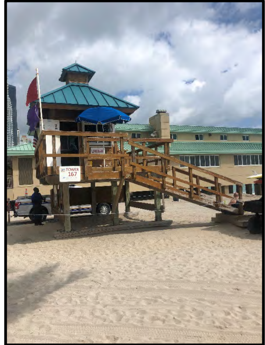
Lifeguard Tower 167 – 16501 Collins Avenue Adjacent to Beach Access 17
