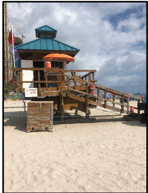
Lifeguard Tower 174 – 17425 Collins Avenue Adjacent to Beach Access 13
