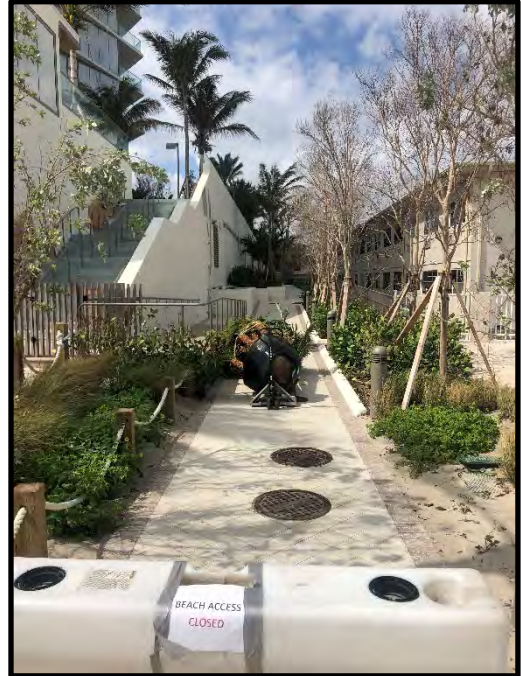
Beach Access 5 – 19051 Collins Avenue Temporarily closed on February 25, 2020
