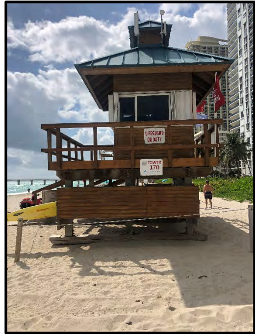
Lifeguard Tower 170 – 17001 Collins Avenue Adjacent to Beach Access 16
