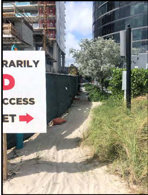
Beach Access 10 – 18555 Collins Avenue Temporarily closed on February 25, 2020
