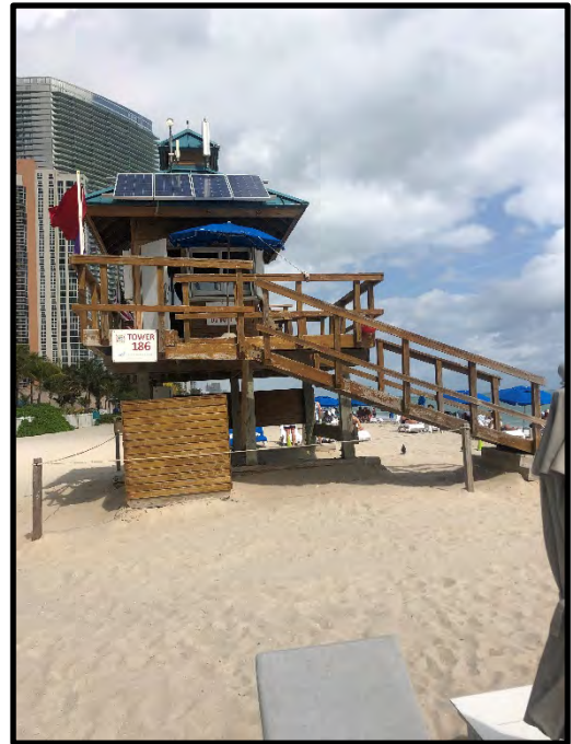
Lifeguard Tower 186 – 18671 Collins Avenue Adjacent to Beach Access 9
