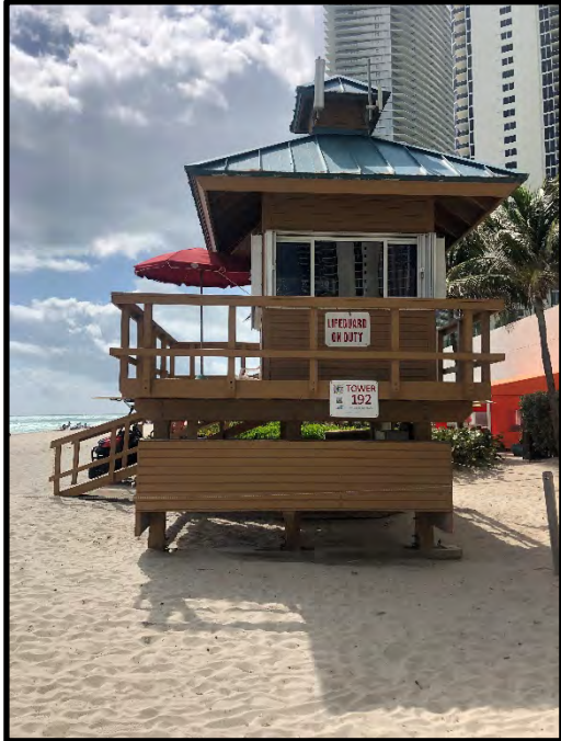
Lifeguard Tower 192 - 19201 Collins Avenue Adjacent to Beach Access 4
