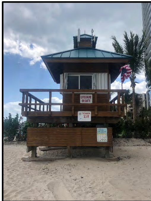
Lifeguard Tower 158 – 16047 Collins Avenue Adjacent to Beach Access 20
