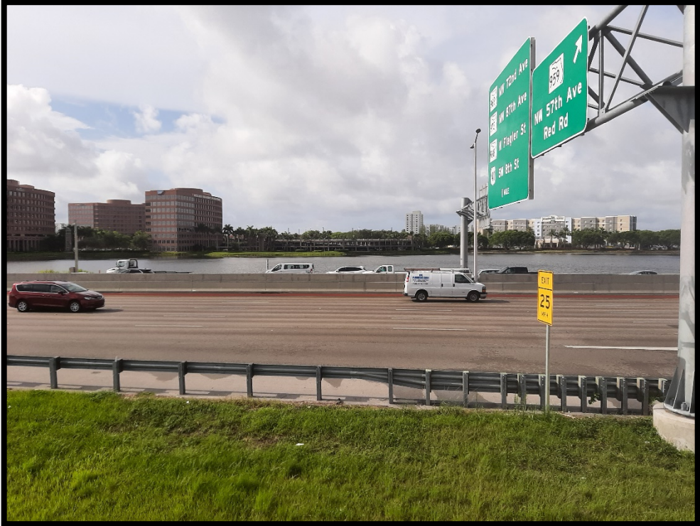
Figure 3.4 South from Perimeter Near Road
