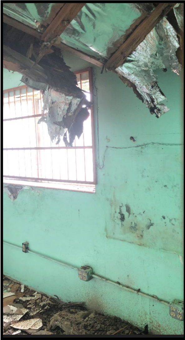
Figure 2.1: Damaged roof
