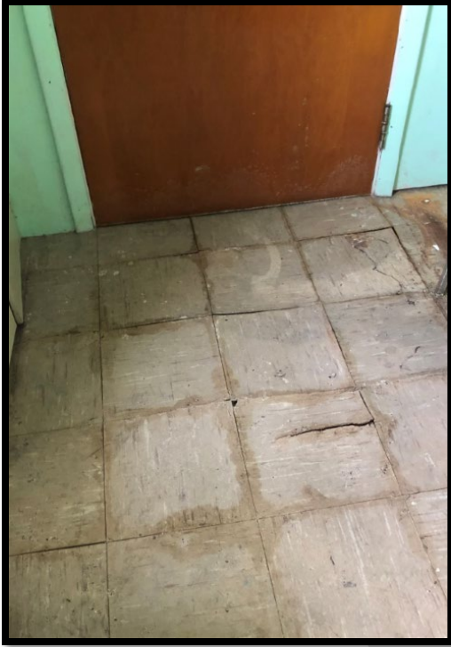
Figure 1.2: Water damage from roof collapse
