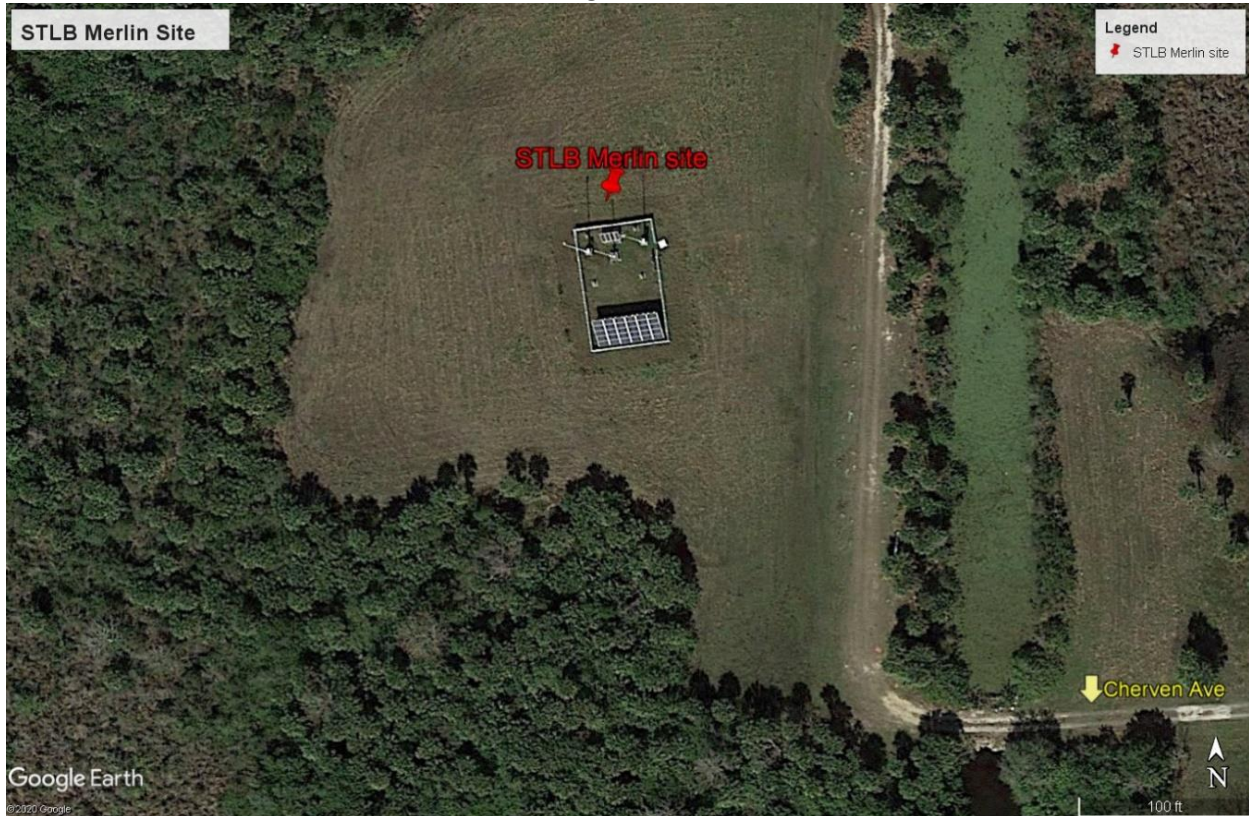
Aerial Image of Leased Area
