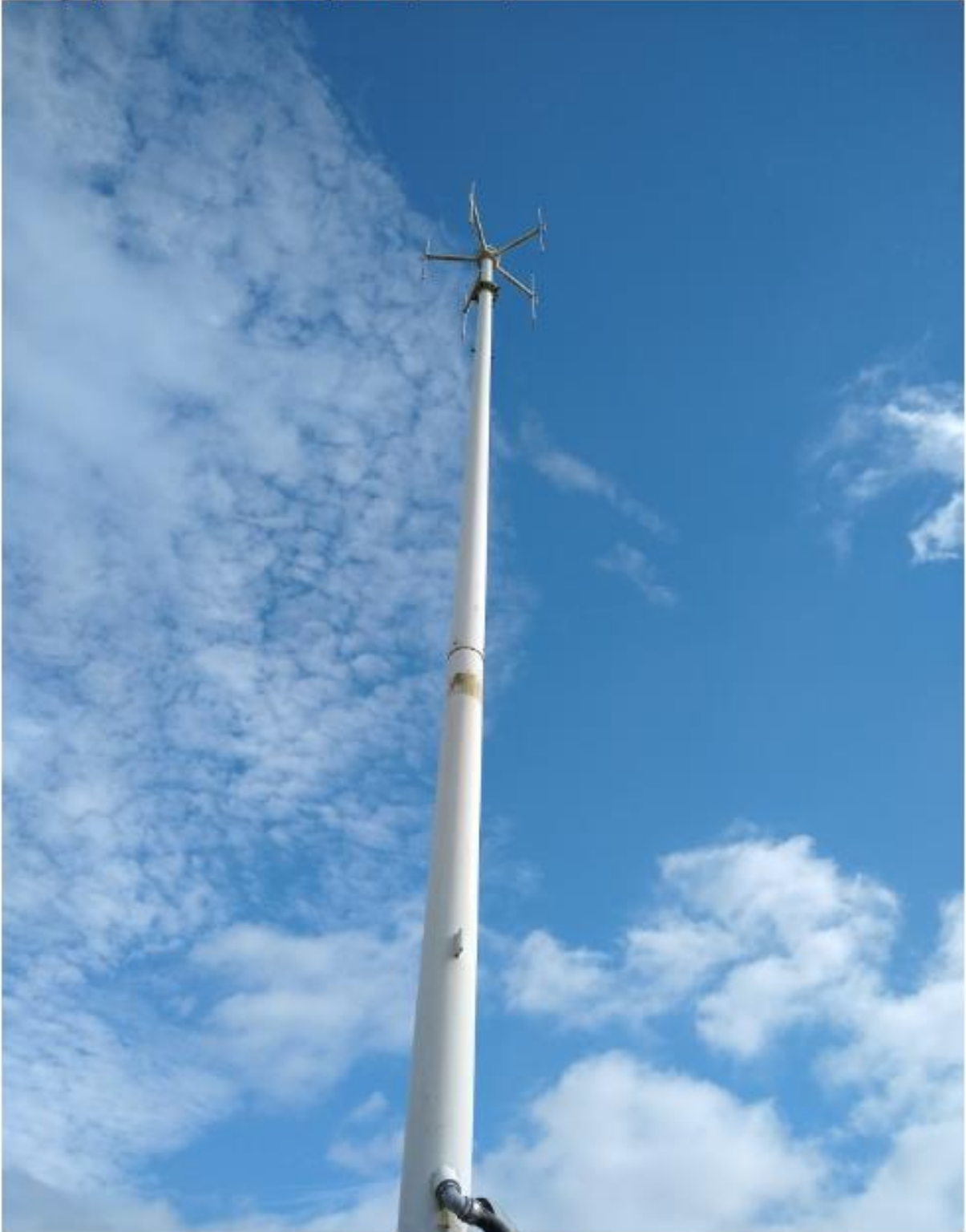
Photographs from 24 SEP 20 Inspection (continued)
