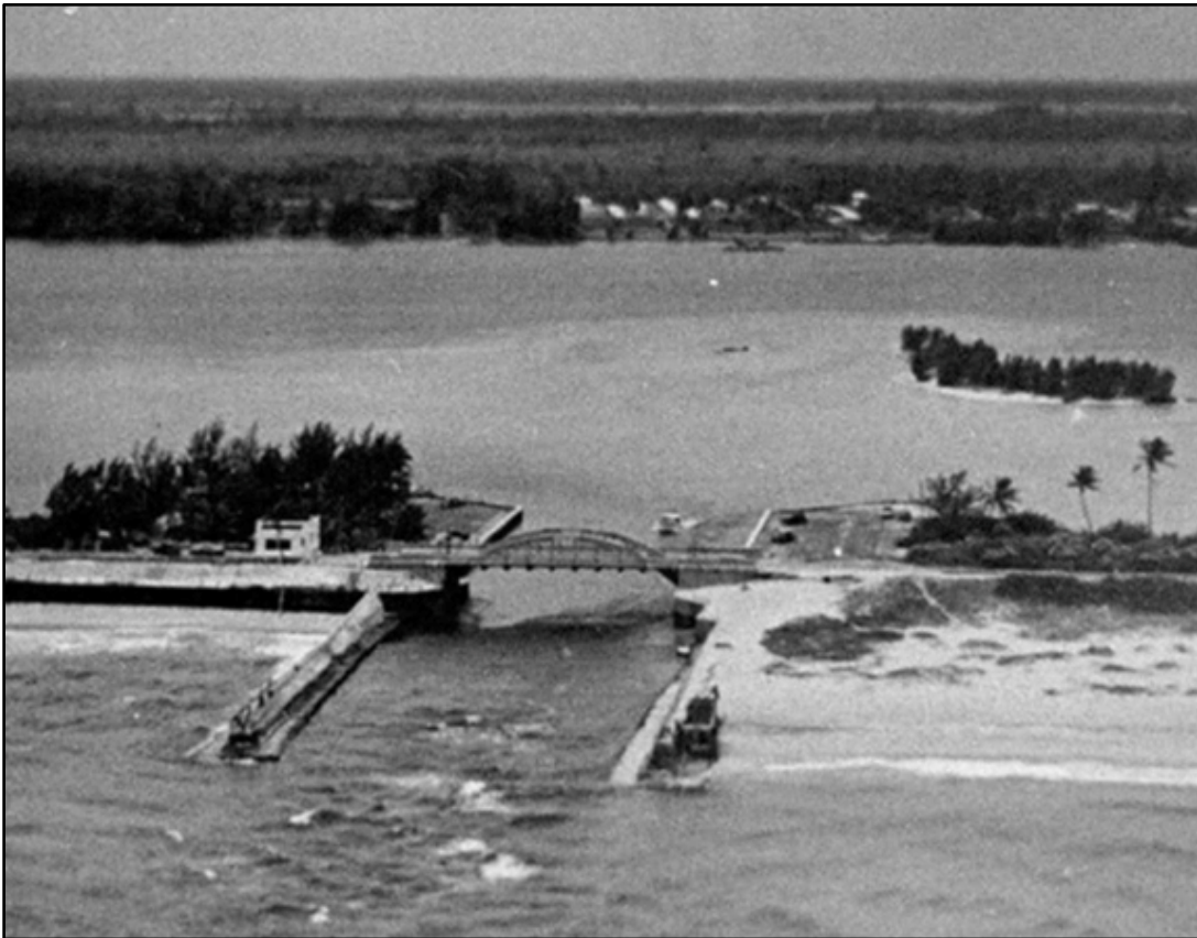
Figure 3. Photo of South Lake Worth Inlet from the 1940's with short straight jetties and the original sand transfer plant. Photo courtesy of the Boynton Beach Historical Society.
