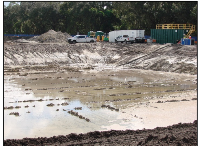
Stormwater pond excavation
