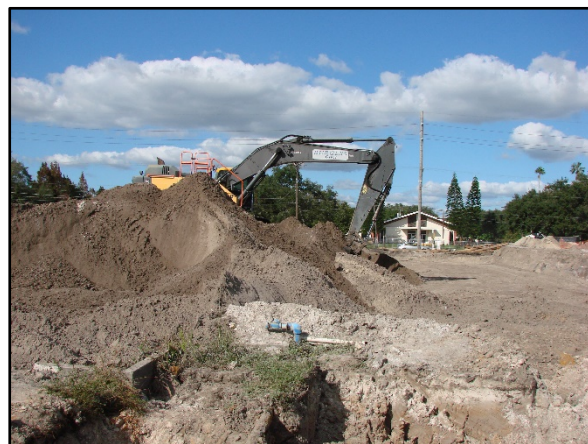
Hanna Avenue City of Tampa offices
