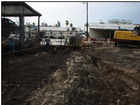
Soil removal by former rail line.
