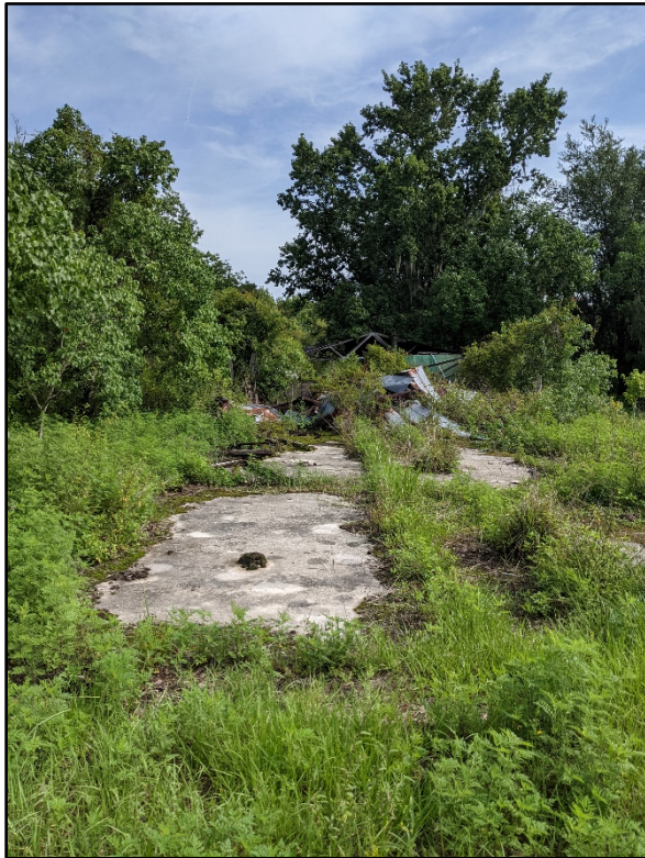
Concrete pad by chicken pens
