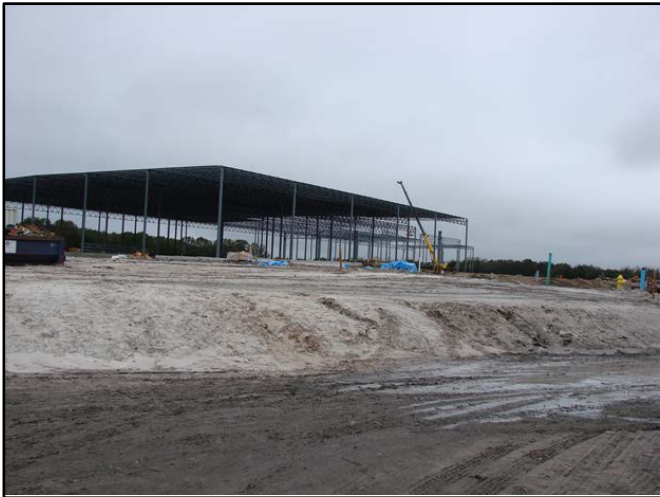
Warehouse construction over fill
