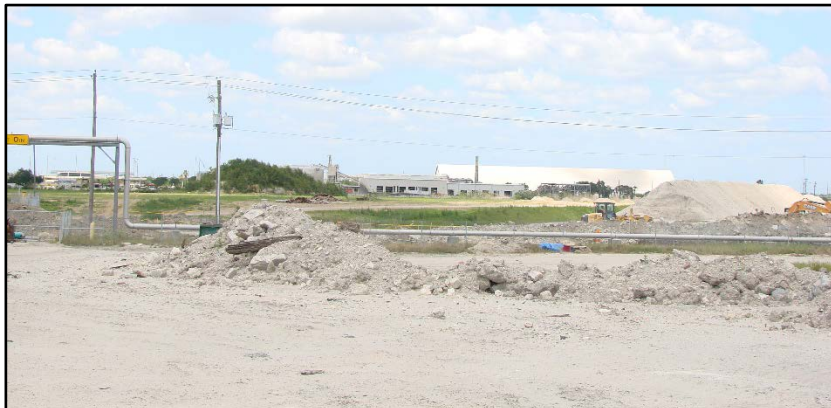
Placement of clean fill at site.
