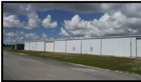
Packaging Facility Prior to Redevelopment
