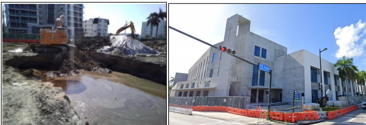
Church under construction
