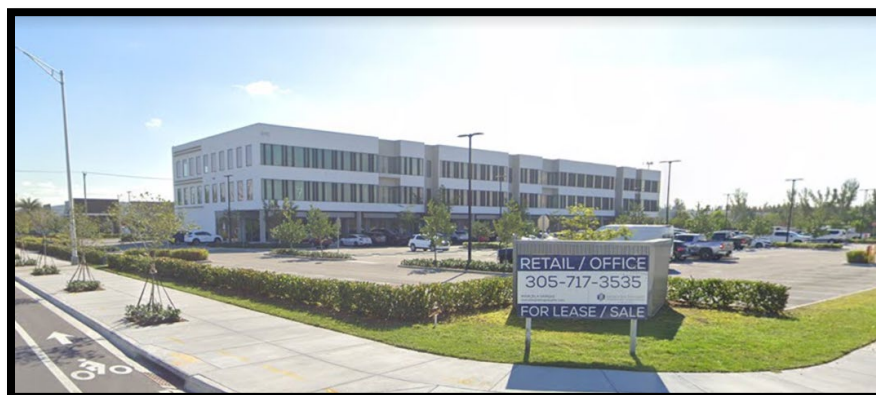
Completed Dolphin Professional Site
