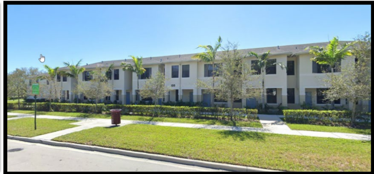
Completed Residential Development
