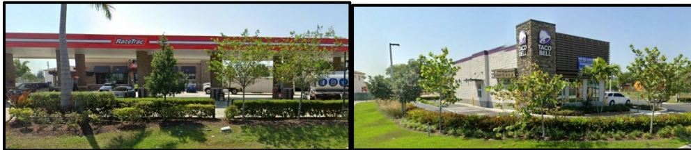
Completed Race Trac and restaurant
