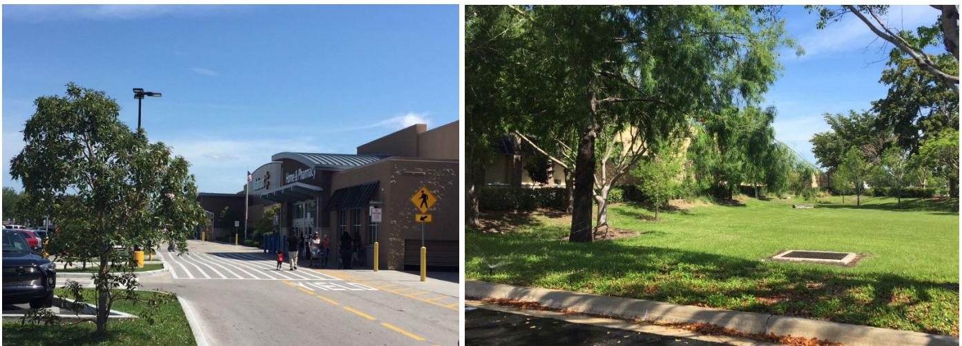
Above Left: The completed Wal-Mart store in Sunrise Above Right: Dry retention area at back of the store
