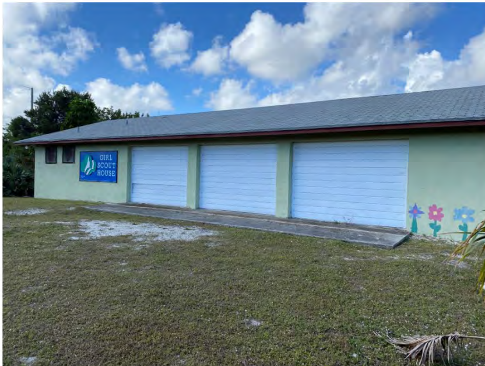
Photo 7 – View of Girl Scout building, facing west.
