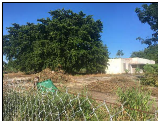
NoMi Square site prior to demolition and redevelopment
