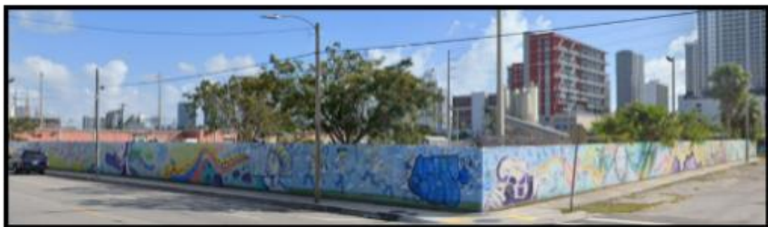
Miami Parcel West Site prior to redevelopment
