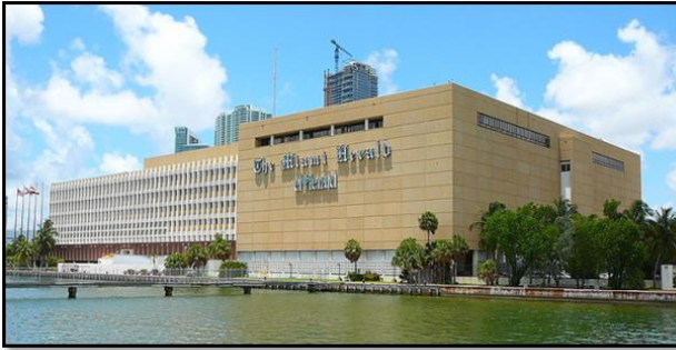
Former Miami Herald Building
