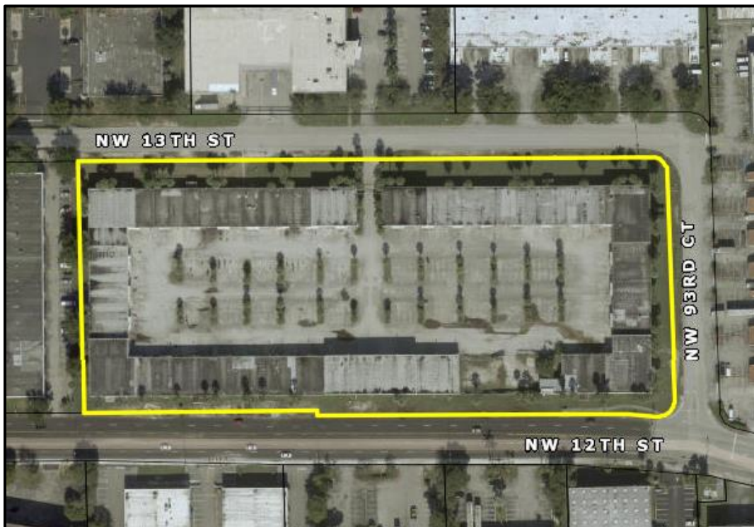
Lithia Motors Green Reuse Site pre-development
