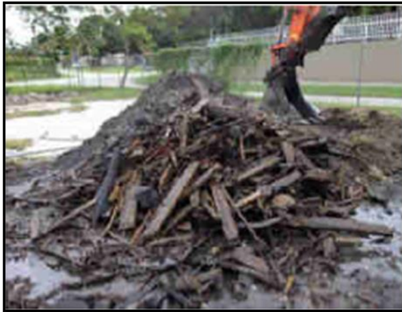
Excavated solid waste
