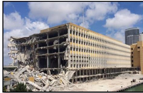
Demolition of Former Miami Herald Building
