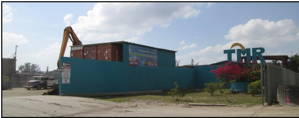
Trademark Metals Recycling Facility
