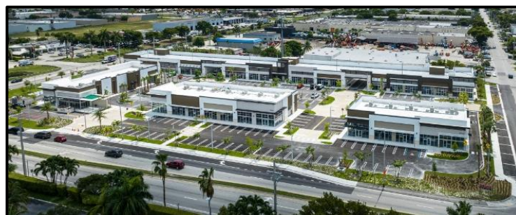
Completed Doral 87 Brownfield Site
