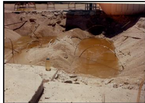
Historic underground storage tank removal (1991)
