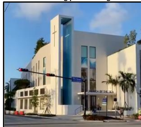
Completed Church By the Sea
