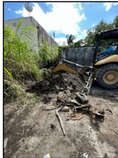
Solid waste documented in test pit
