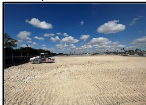
Site cleared for redevelopment
