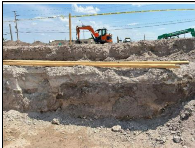
Soil profile during foundation construction
