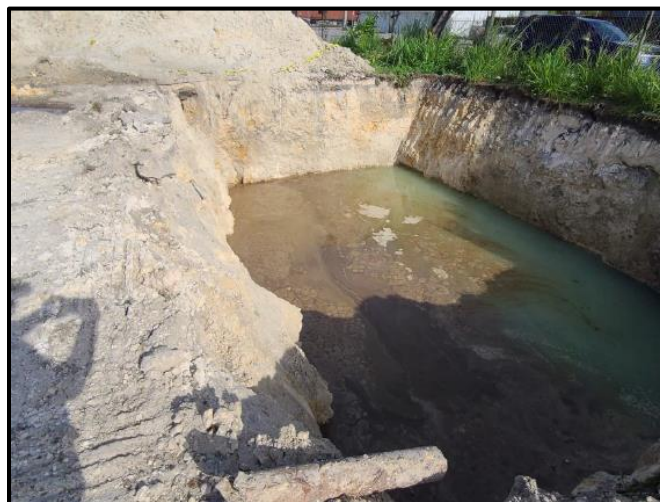
View of excavation 6/15/2023 at the McArthur Dairy Site
