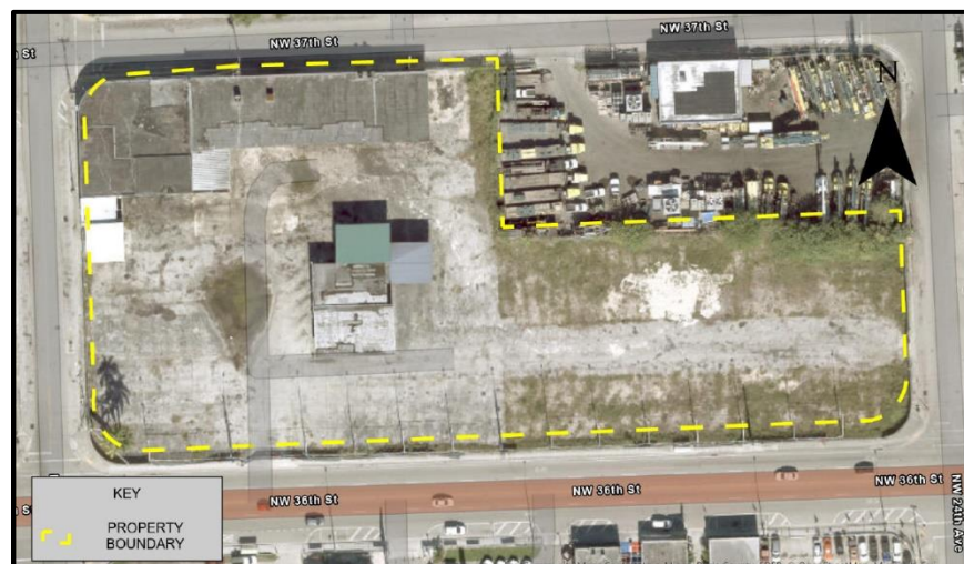
Bindi Investments Site pre-redevelopment
