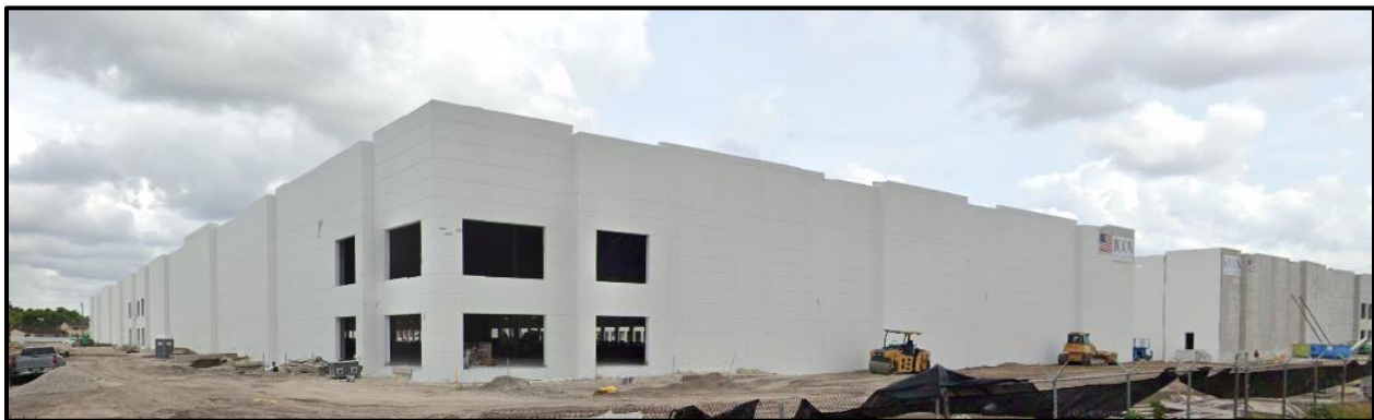
Construction of Warehouse Development
