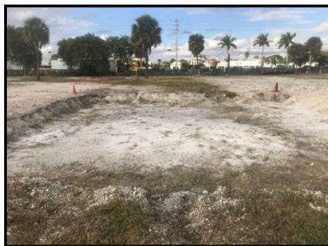
Excavation at the site
