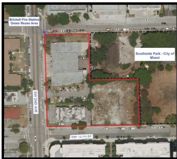
Brickell Fire Station Site prior to redevelopment
