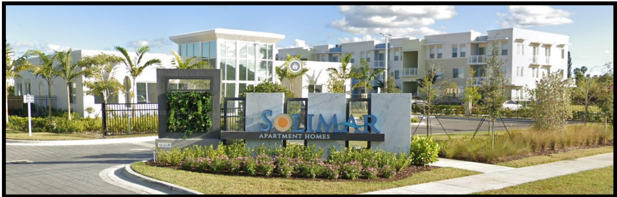
Completed Solimar Apartments
