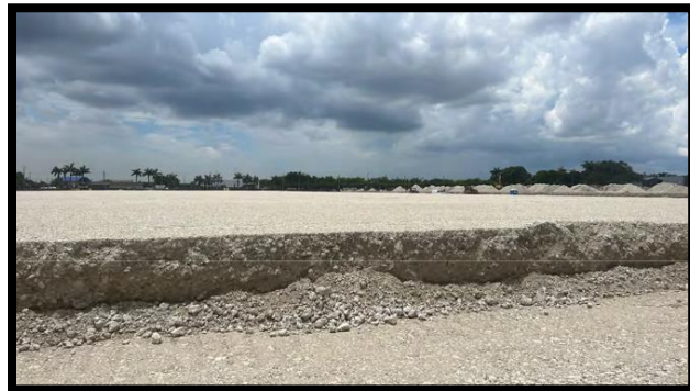
Construction of the engineering control cap
