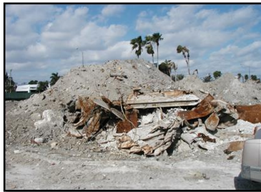
Solid Waste excavated
