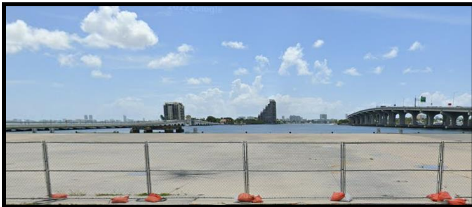
Resorts World Site after demolition and prior to redevelopment
