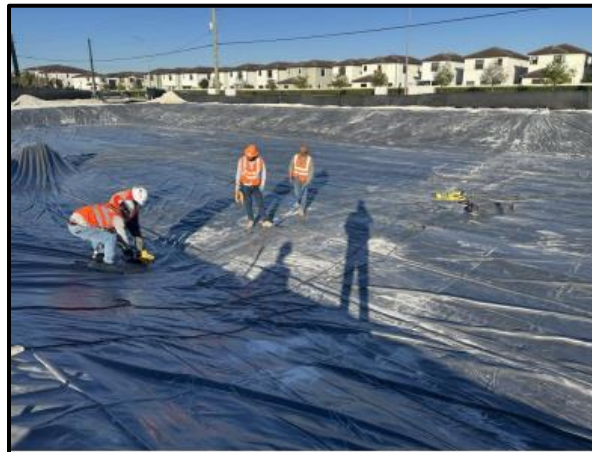
Liner installed in retention area
