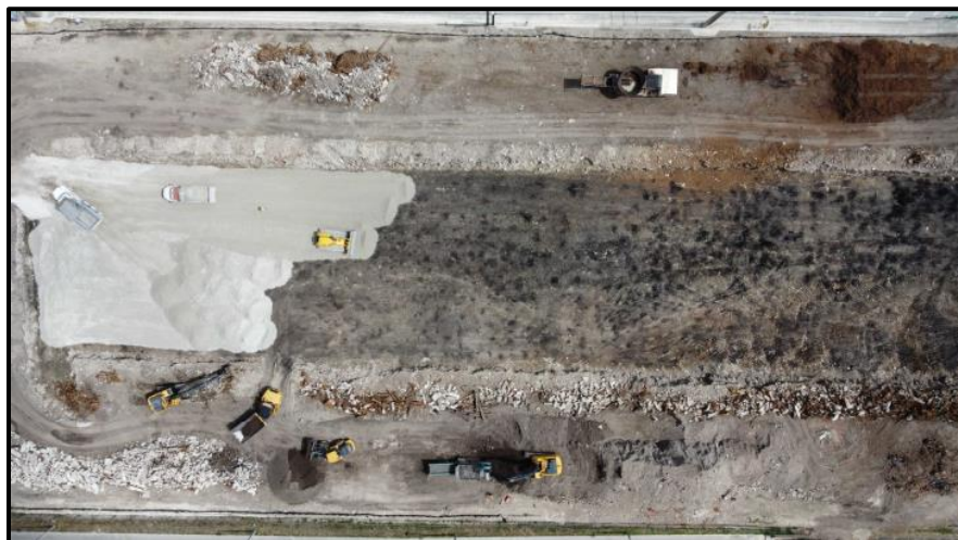
Recovered Screened Material screening and import of crushed concrete during development
