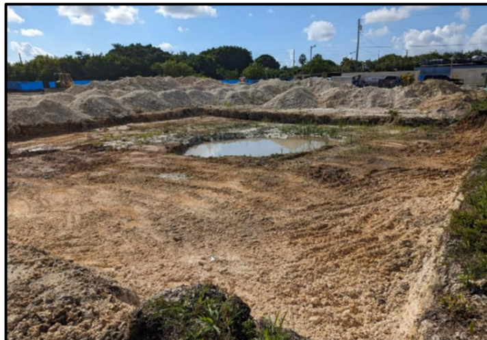
Excavation at the site
