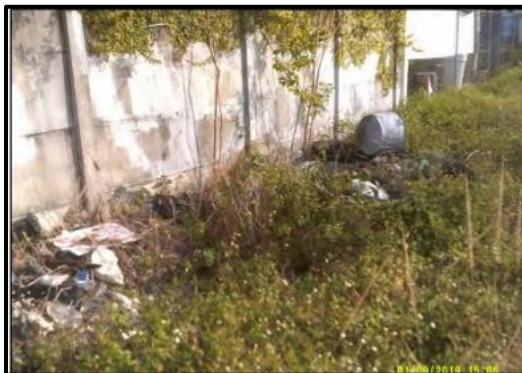
Debris noted along abandoned railroad corridor
