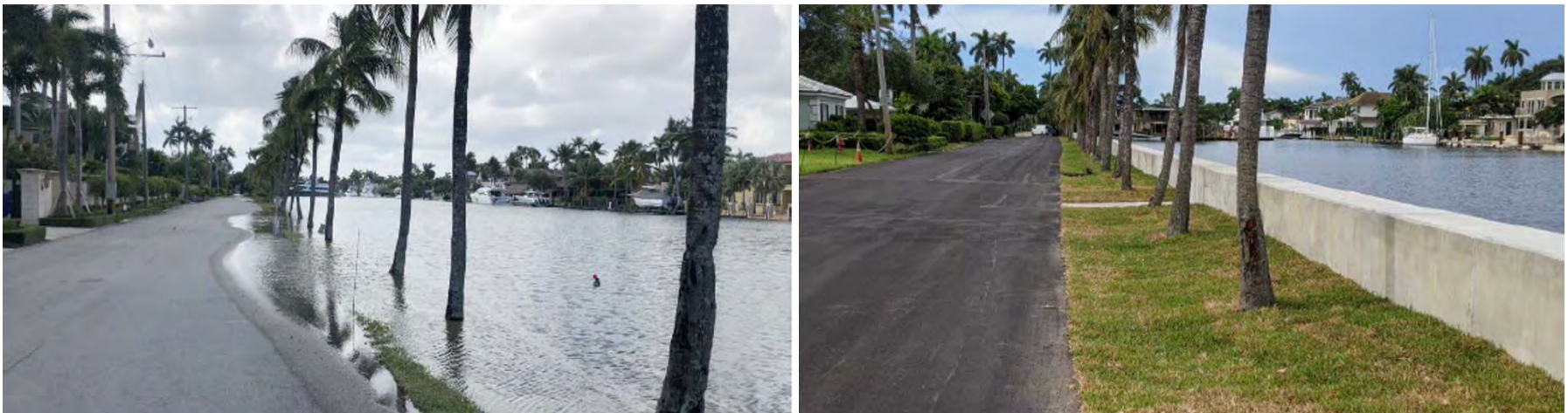
Figure 22. Before and after seawall improvements along Isle of Palms Drive, Fort Lauderdale. (Photo credit: City of Fort Lauderdale)
