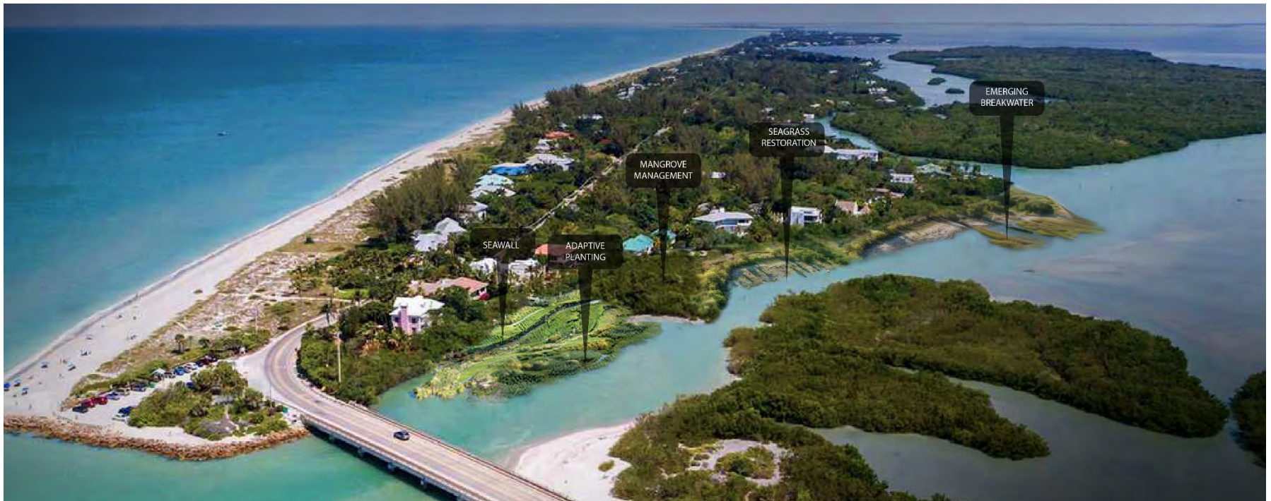
Figure 23. Potential adaptation strategies are illustrated on a drone image in Captiva Island to help stakeholders visualize possible coastline enhancements and guide the selection of appropriate strategies. (Rendering credit: Sasaki )
