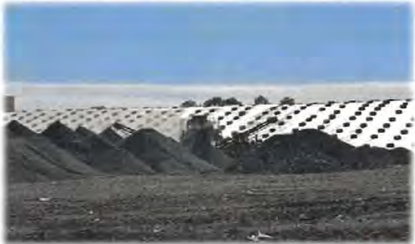
Figure 6-2 Segregated Aggregate Piles
