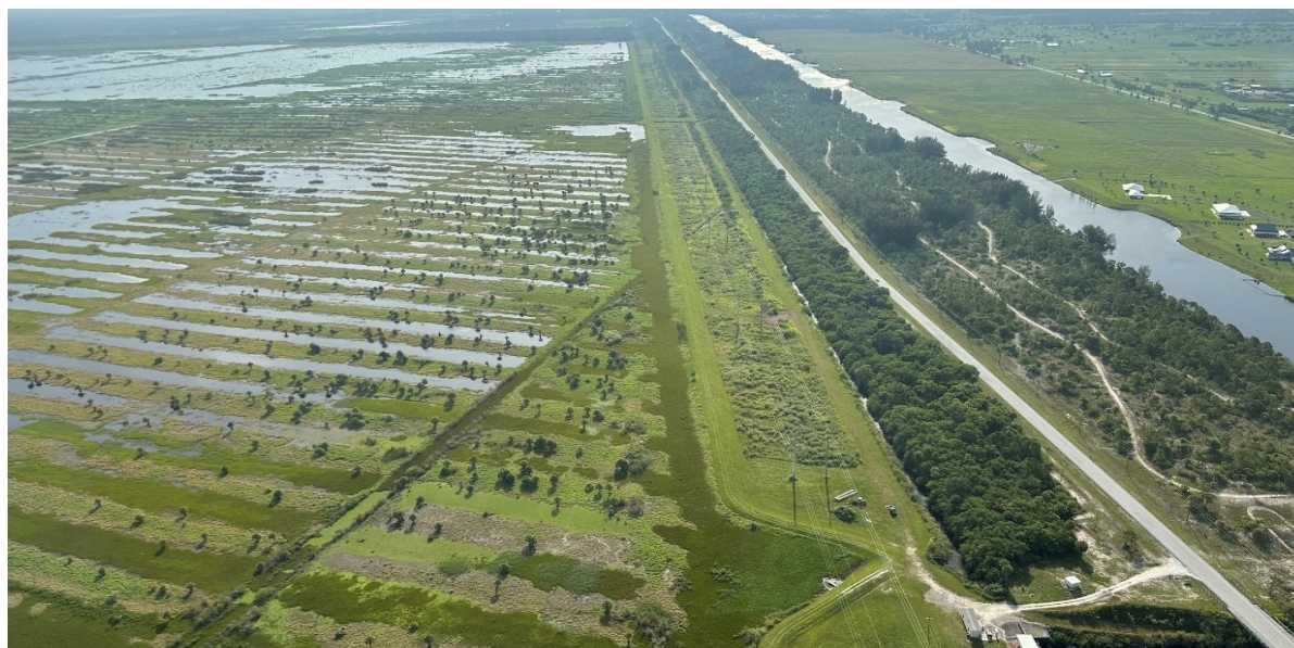
Caulkins Water Farm Project, Martin County
