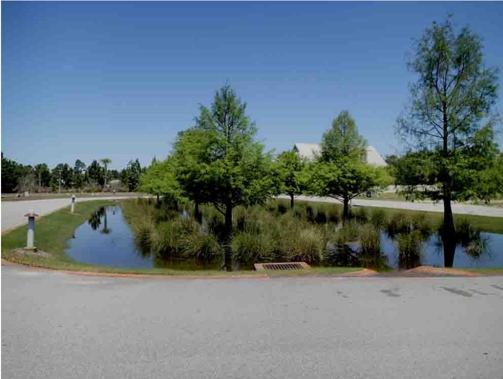
Photo of stormwater pond onsite. Native pond cypress and native cordgrass were planted in a seasonally flooded stormwater pond.
