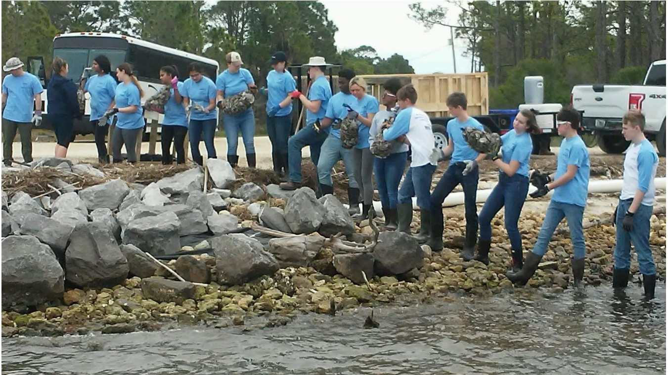
Photo 19 / Volunteers in action – building the Sawyer St. living shoreline.
