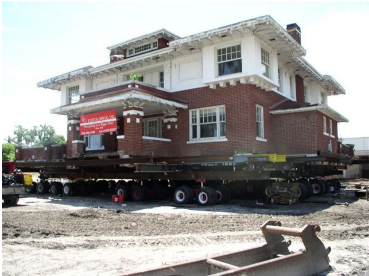
Photo Credit: Flint and Doyle Structural Movers
