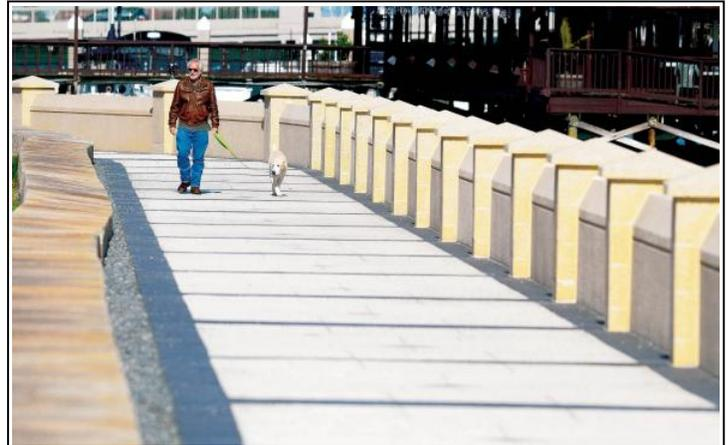
*This photo shows what remains of the historic seawall, to the left, and the new taller seawall, to the right, with the two seawalls separated by a walking path.<sup>42</sup>*
