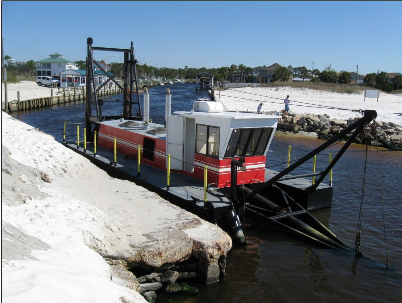
Figure 21: Mexico Beach Inlet being dredged to bypass material to Mexico Beach, photo by Ralph Clark (DEP) in April 2010.
