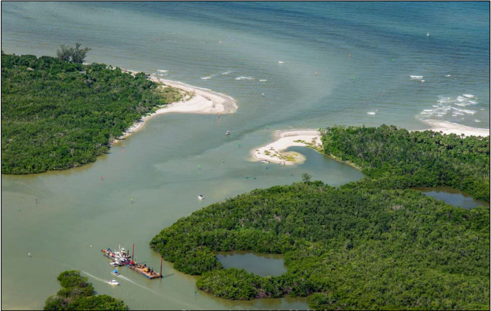
Figure 25: Wiggins Pass being dredged to bypass material to the north and south. Photo courtesy of Humiston and Moore, July 2018.
