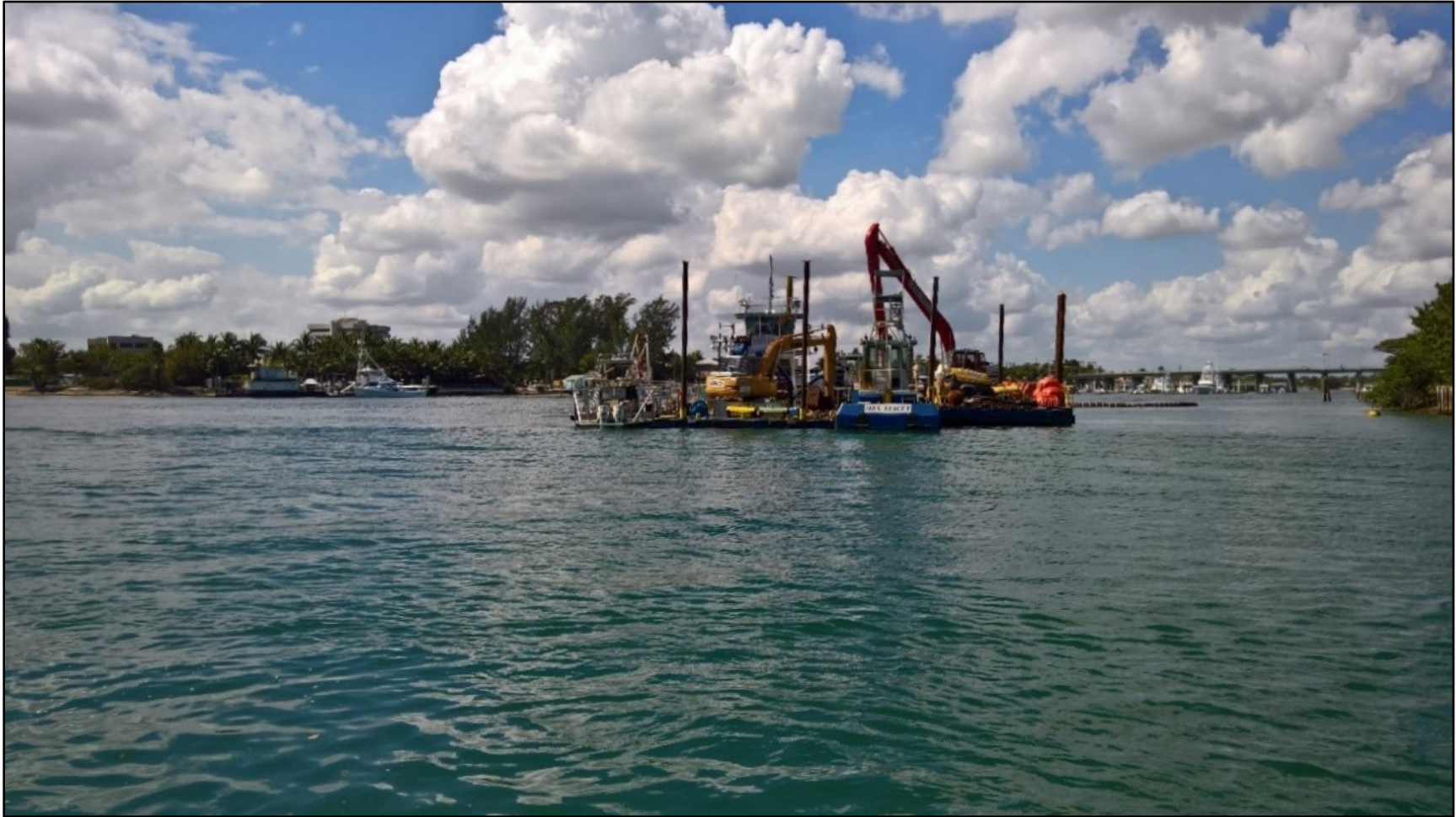
Figure 13: Jupiter Inlet with the Cavache Dredge working within the inlet to bypass sand, March 2017. Photo by Libbie McDearnid (DEP) in March 2017.
