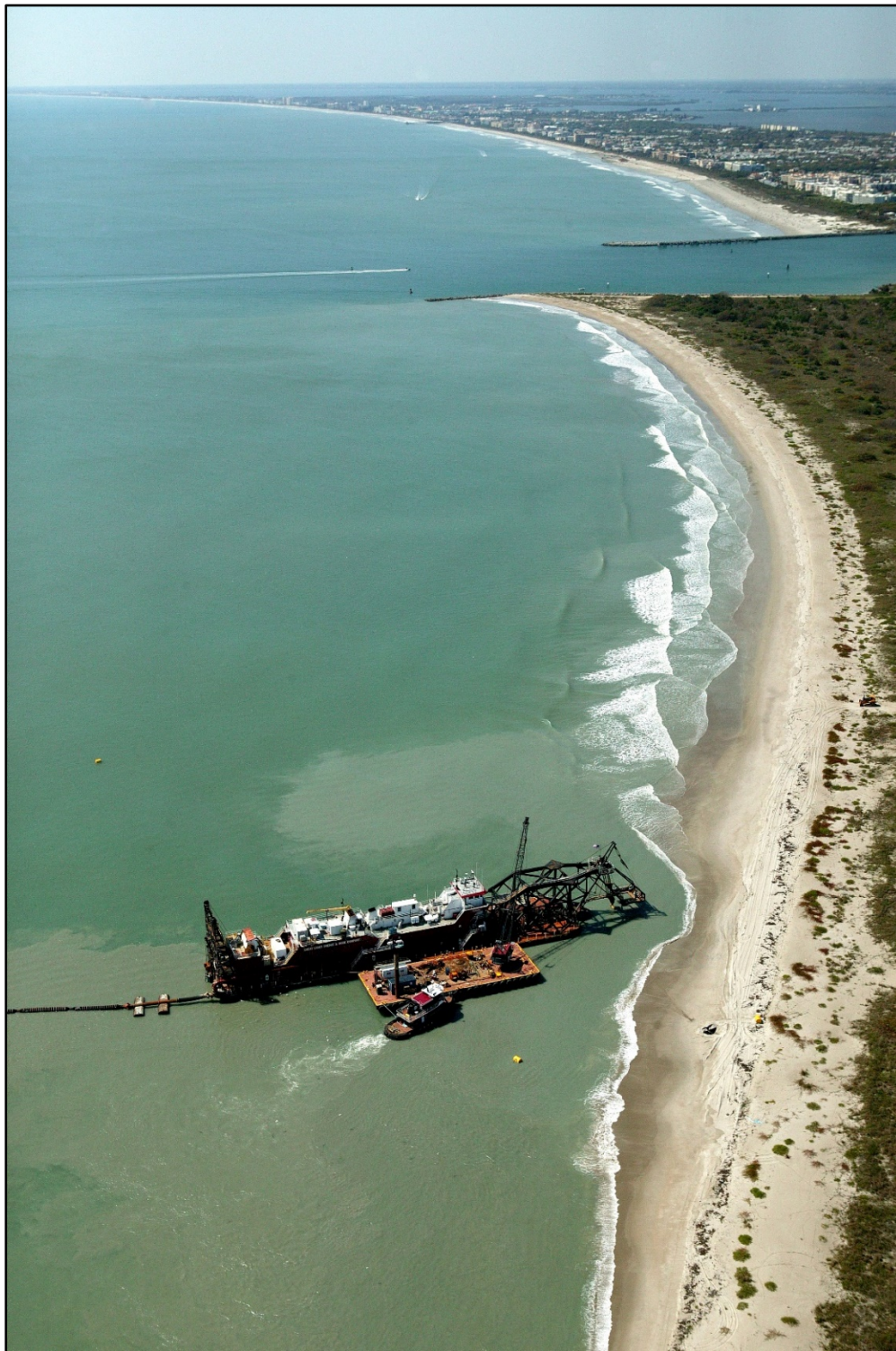
Figure 7: A cutter suction dredge north of Canaveral Inlet dredging sand from the nearshore to be bypassed south to the City of Cape Canaveral and Cocoa Beach. Photo courtesy of Olsen Associates, March 2010.
