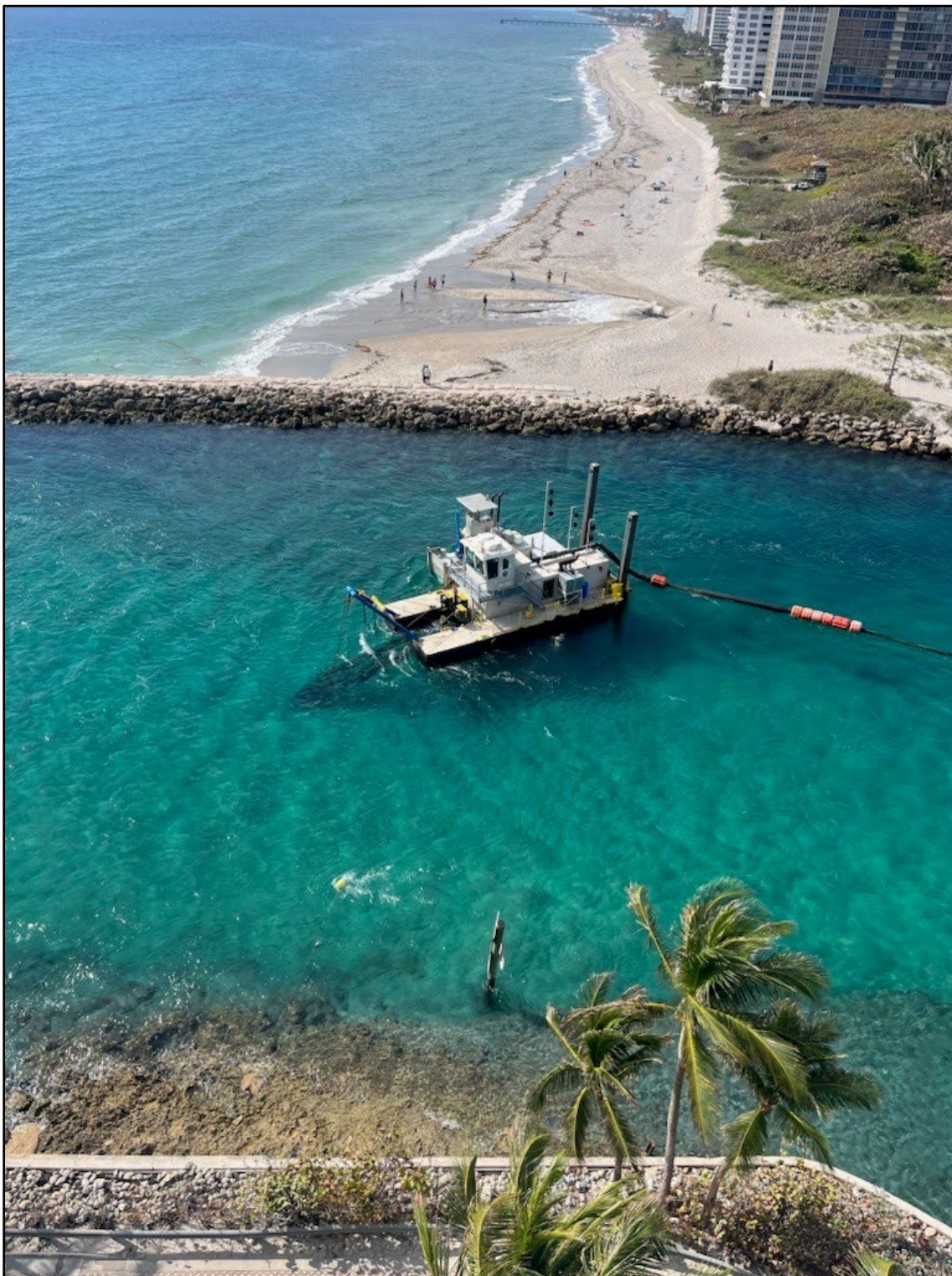
Figure 13. Boca Raton Inlet with City dredge bypassing sand south of the inlet. Photo courtesy of the City of Boca Raton - Zach Bihr, March 2024.
