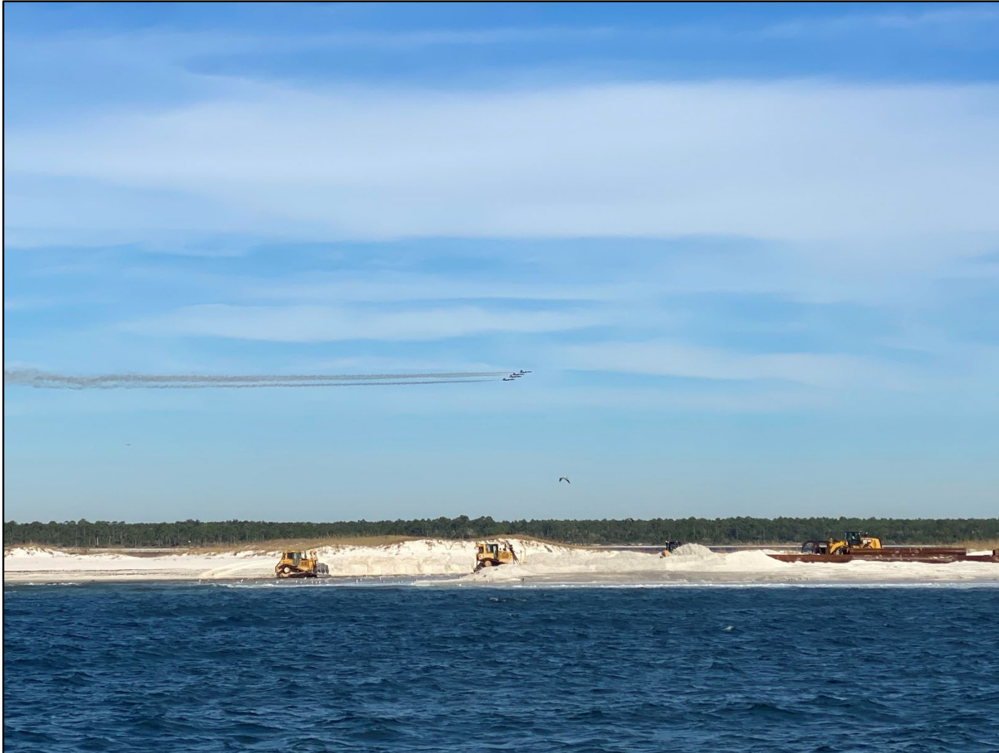
Figure 21. Pensacola Pass Federal Navigation Channel dredged to place material at Johnson Beach in Gulf Islands National Seashore Park on Perdido Key. Photo courtesy of Timothy Day with Escambia County, November 2024.
