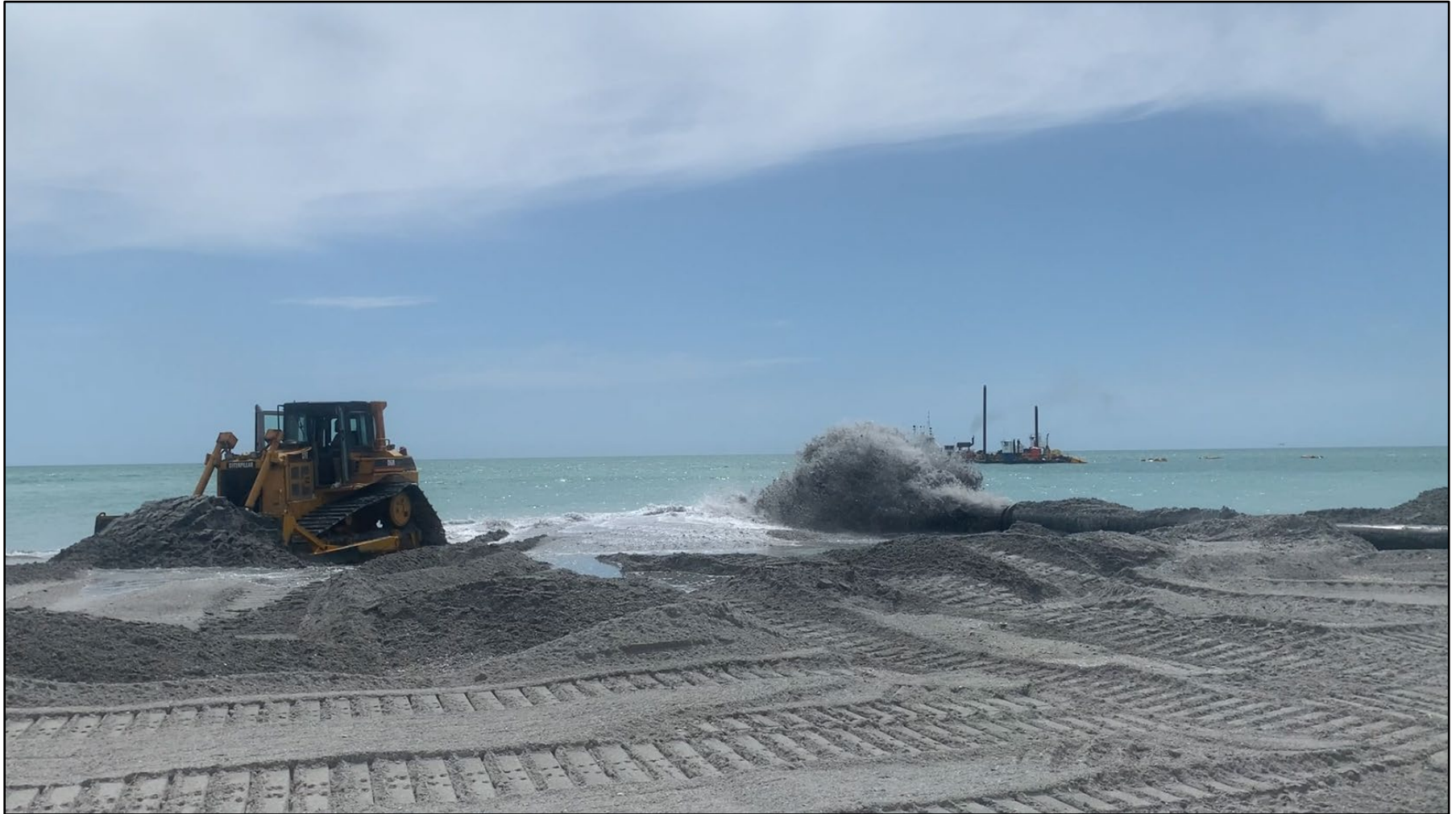
Figure 26. Sand bypassing from Stump Pass navigational channel/ebb shoal with material being placed along the Palm Island development on Knight Island. Photo courtesy of Michael Poff, P.E., Coastal Engineering Consultants, May 2025.
