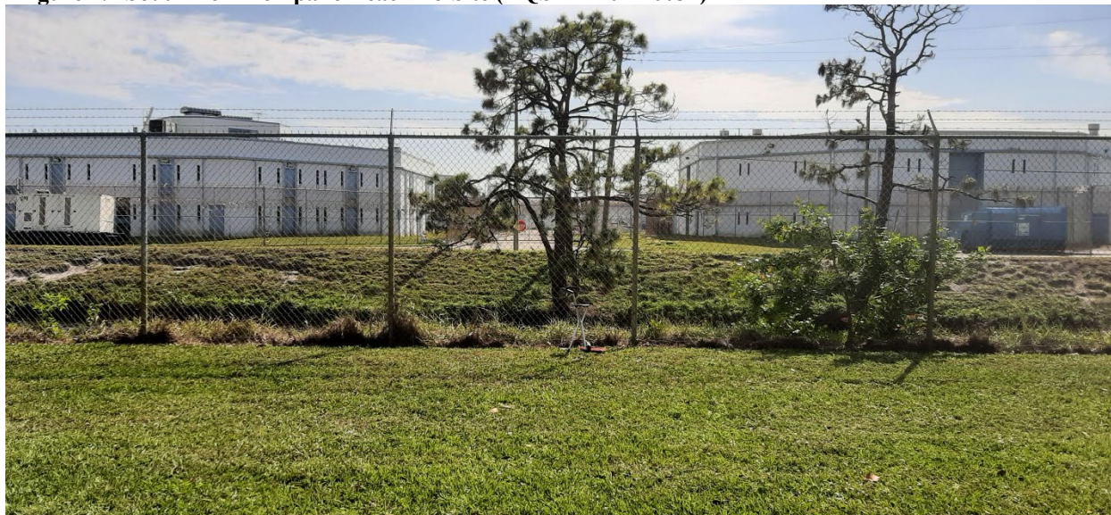
Figure 7.4 South from Pompano Beach EJ Site (AQS # 12-011-0037)
