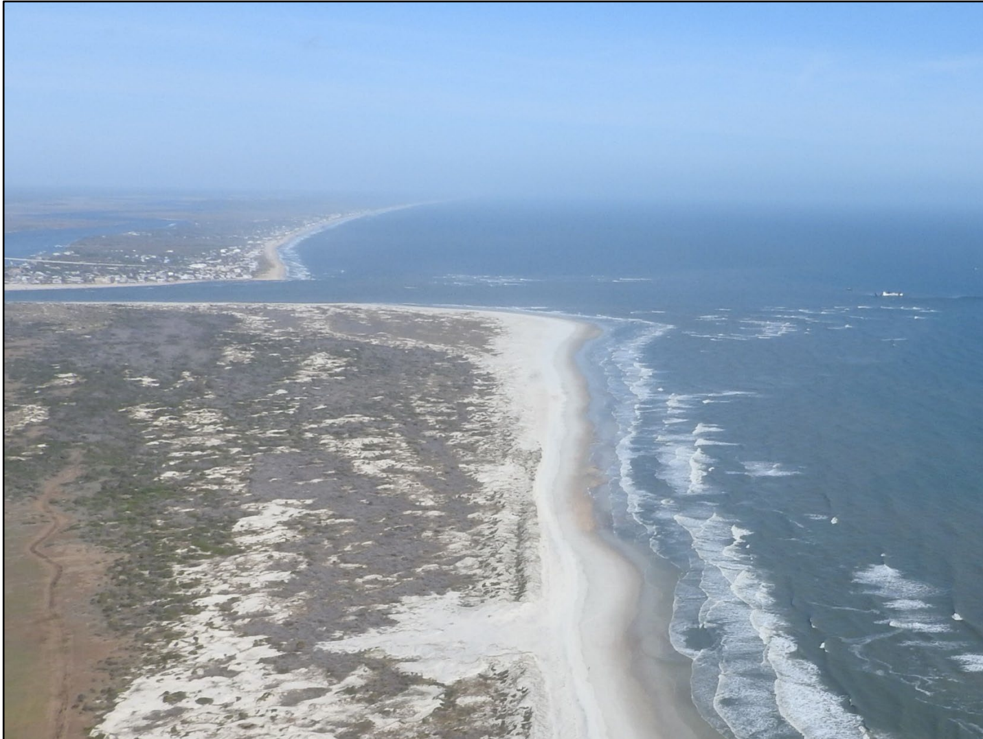
Figure 1: St. Augustine Inlet ebb shoal being dredged to bypass material south to construct the St. Augustine Beach nourishment project. Photo by Guy Weeks (DEP), February 2018.
