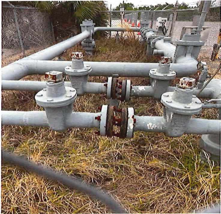
TECO Gas Lines To Facility
