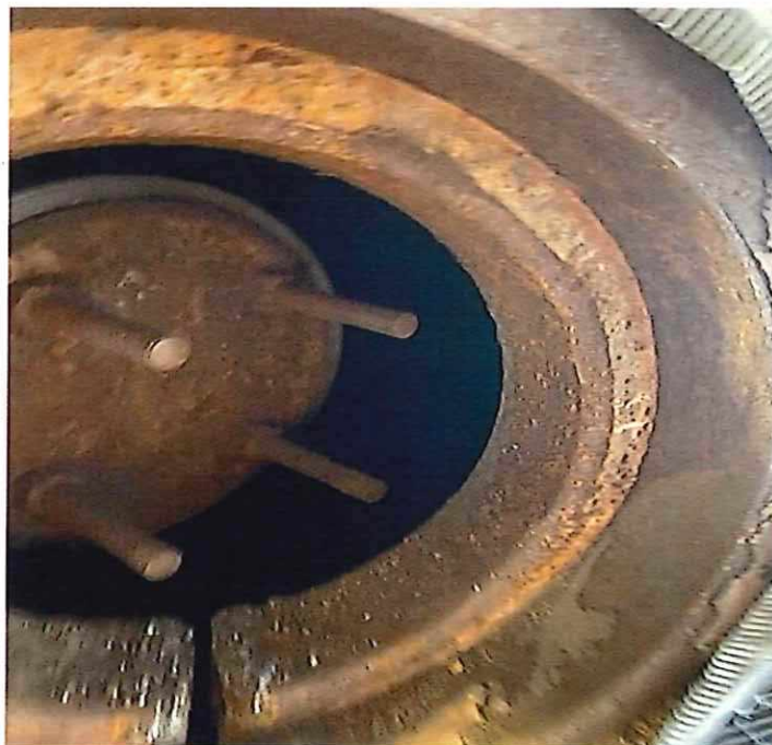
No. 3 Power Boiler Steam Drum Open and Cut
