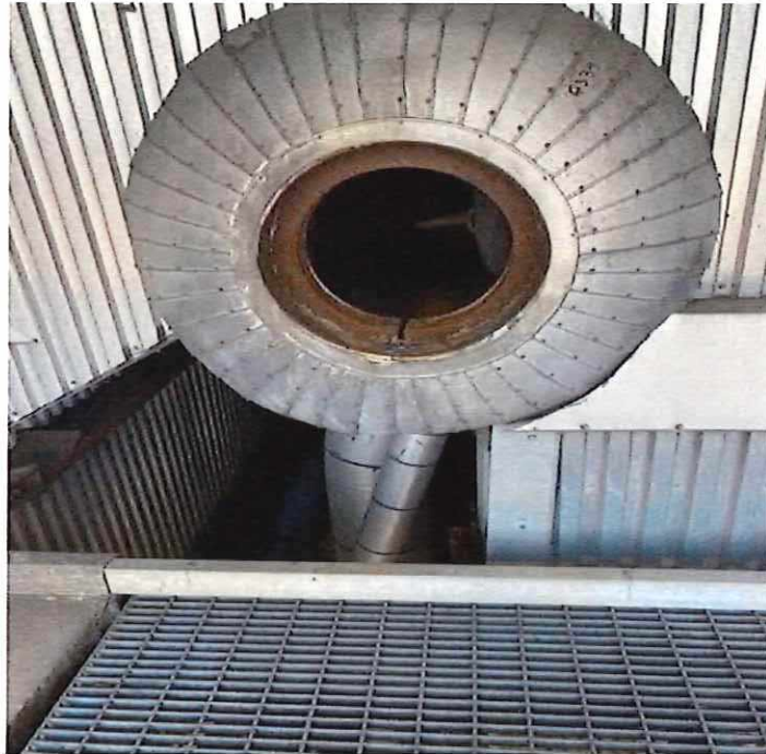
No. 3 Power Boiler Steam Drum Open and Cut
