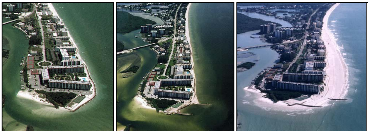
Figure 4. North end of Bonita Beach before construction of the terminal groins (left), after construction of the terminal groins (middle), and after placement of 217,000 cy of sand (right) (Olsen, 2023).
