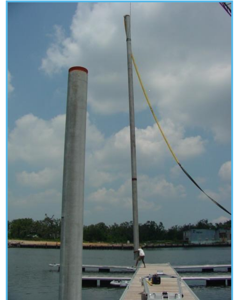
70' piling being installed
