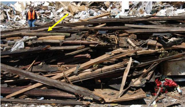
*Loads from the demolition of outdoor structures will typically contain CCA-treated wood. Pole at the upper left is treated.*
