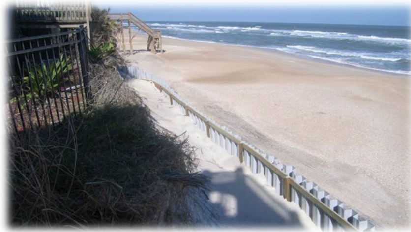
Figure 3 Under CCCL emergency permit procedures, beachfront property owner can install temporary wooden retaining walls, cantilever sheet pile walls (without caps, tiebacks, or other reinforcement), or sand bags (less than 100 pounds each).
