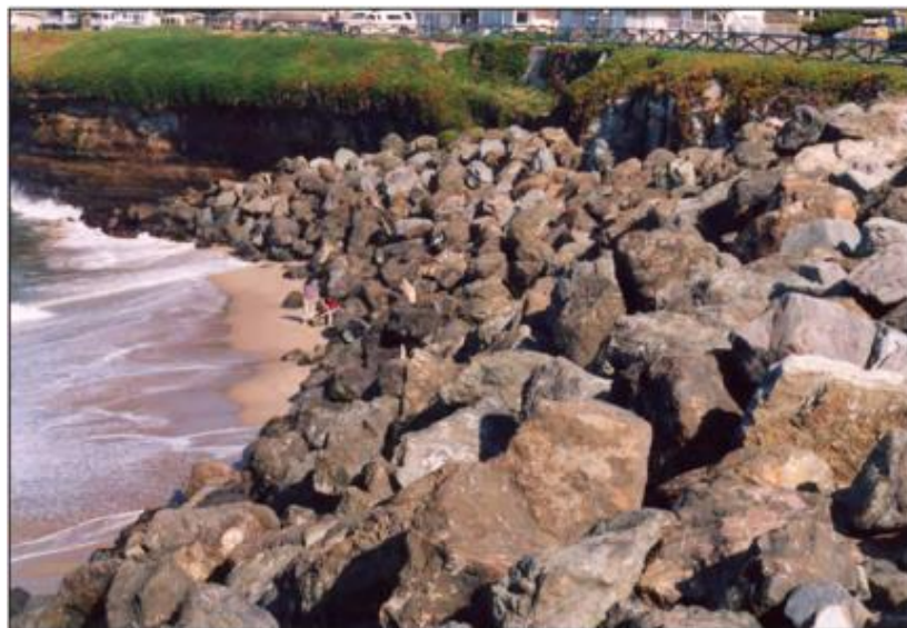
Figure 1. Revetment in Santa Cruz, California (note the absence of a sand beach). 8
