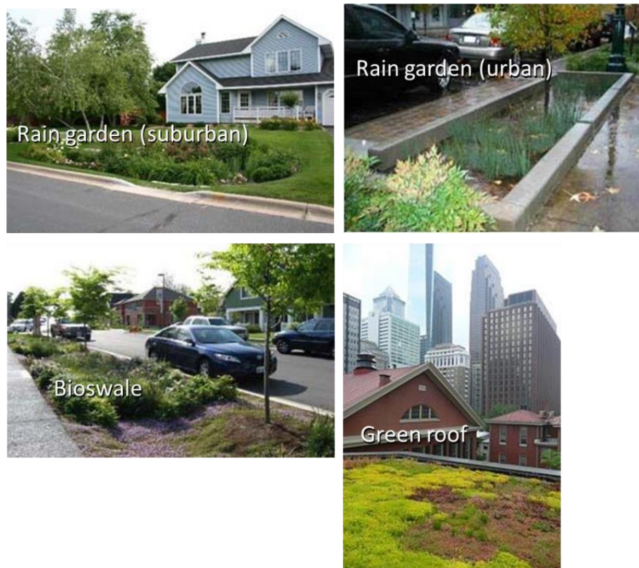
Figure 8. Illustrations of installed LID/GI. 59
