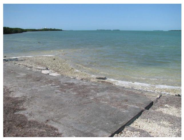
Uneven surfaces such as this one at the end of a ramp can be difficult for wheelchairs to navigate. Concrete ramps are also known to be slippery.
