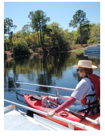
This type of floating dock with rails and a launch chute has received high praise from those with physical challenges. The rollers can sometimes become gummed up, so occasional maintenance may be required. Installation is similar for that of any floating dock.
