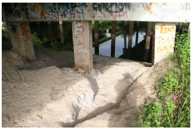
Unimproved launches such as this unofficial access point beneath a bridge can be problematic for anyone, and can promote erosion. Steps and crushed stone would be two ways to improve this situation, or a different site nearby could be developed.
