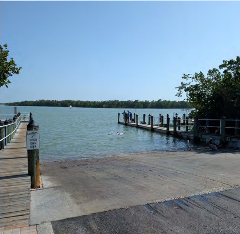
Access at Goodland Boat Park
