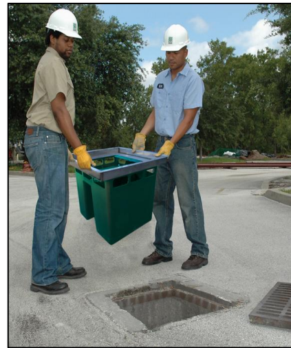
Example of Catch Basin Installation Source: Interstate Products, Inc.
