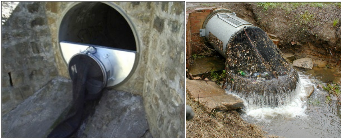
Example of Netting Trash Strap Installed in Stormwater Pipe Source: Stormwater Systems, Inc. 2019
