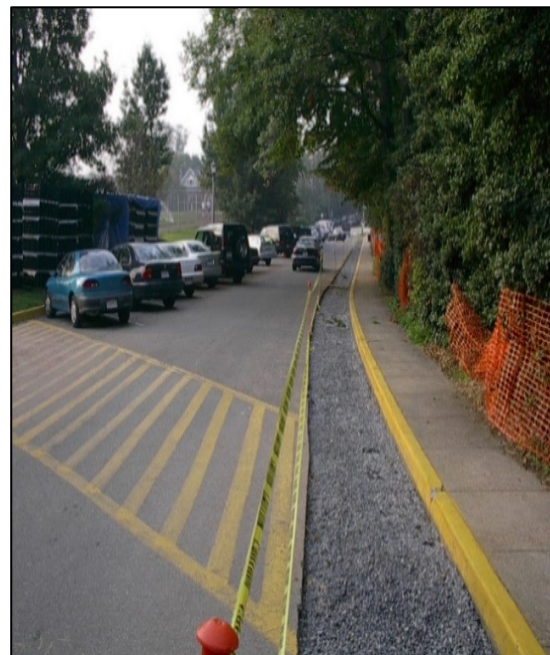
Example of Infiltration Trench Being Constructed along the Edge of a Street
