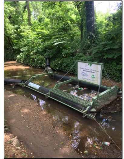
Example of a Stormwater Systems, Inc Trash Trap Source: Stormwater Systems, Inc. 2019
