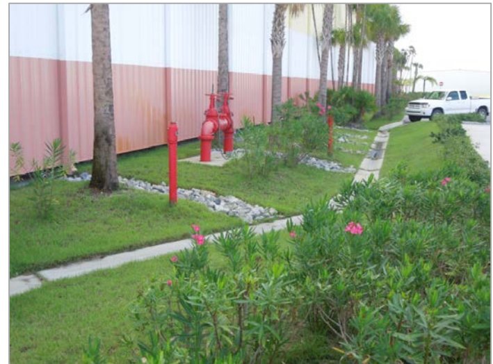
Bluepoints Marina, Cape Canaveral, FL
