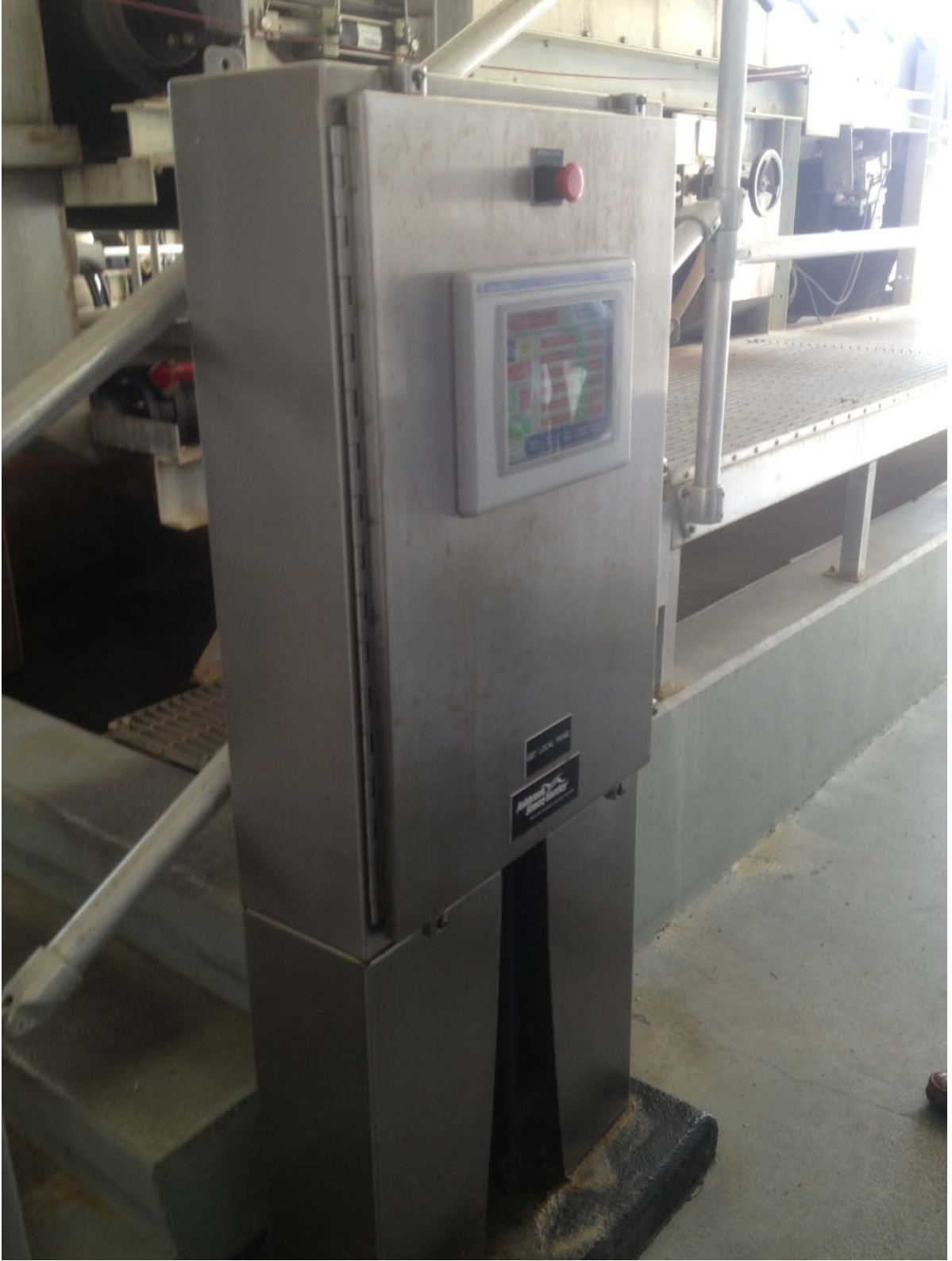
Exhibit No. 11 – Existing GBT Local PLC Panel at the NEWRF
