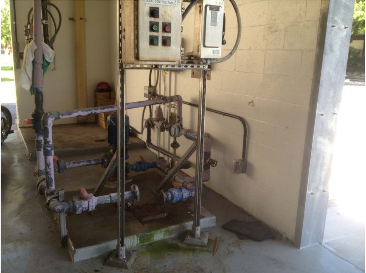
Exhibit No. 7 – Existing GBT Wash Water Pumps at SWWRF
