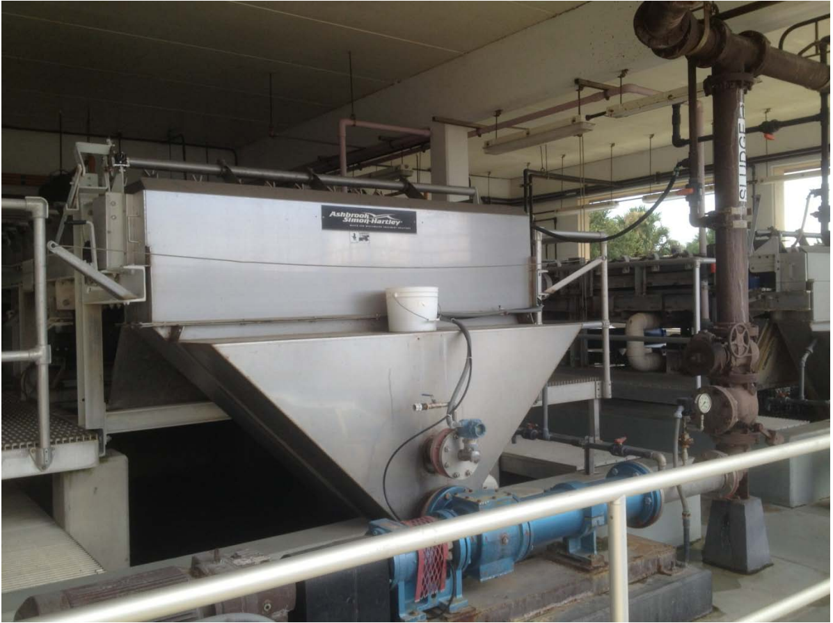
Exhibit No. 10 – Existing GBT with Thickened Sludge Transfer Pump at the NEWRF
