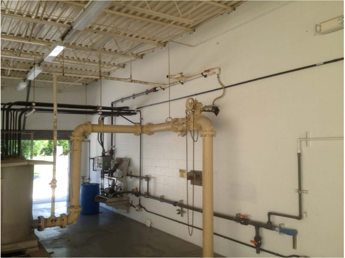
Exhibit No. 14 – Existing Polymer Injection System at the SWWRF
