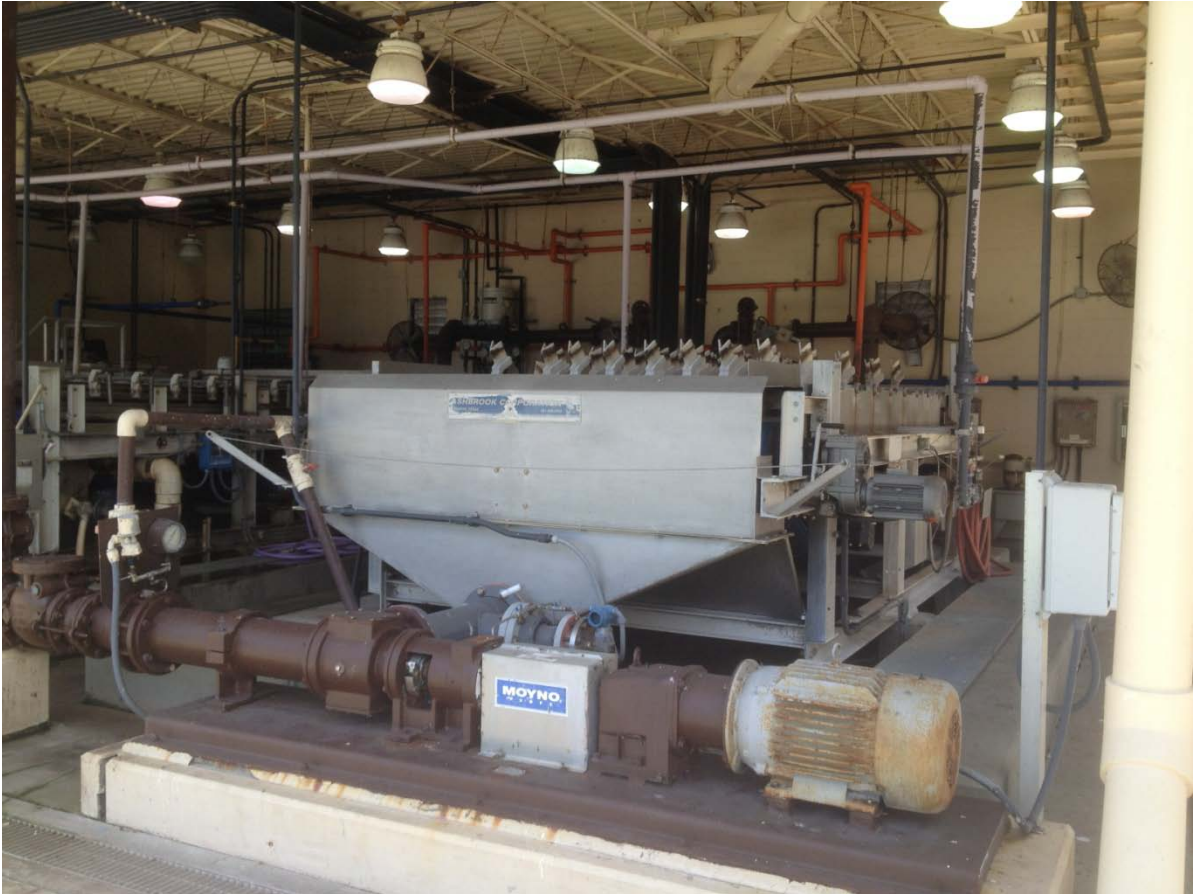
Exhibit No. 8 – Existing GBT with Thickened Sludge Transfer Pump at the NWWRF
