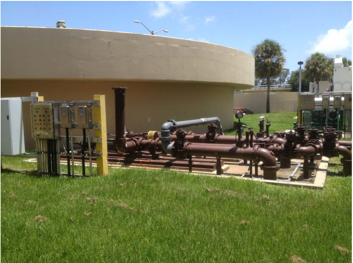
Exhibit No. 4 – Existing GBT Feed Progressive Cavity Pumps at SWWRF
