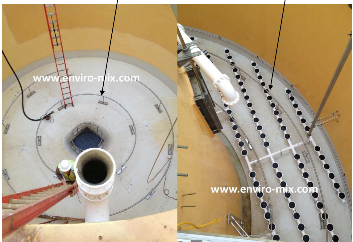
Figure 4.3 Photo Schematic of “Large-Bubble” Mixing Systems for Sludge Holding Tank
