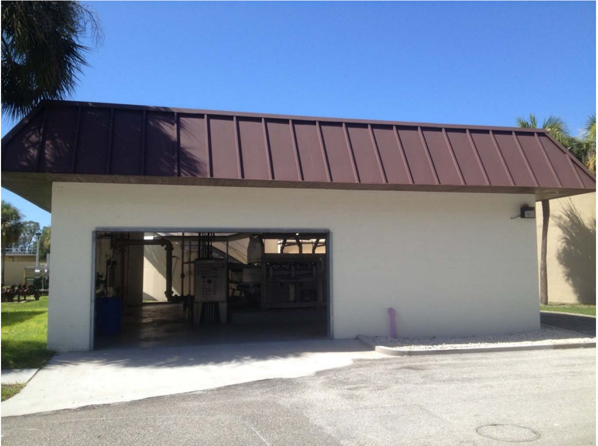
Exhibit No. 1 - North Elevation View of Existing Sludge Thickening Building
