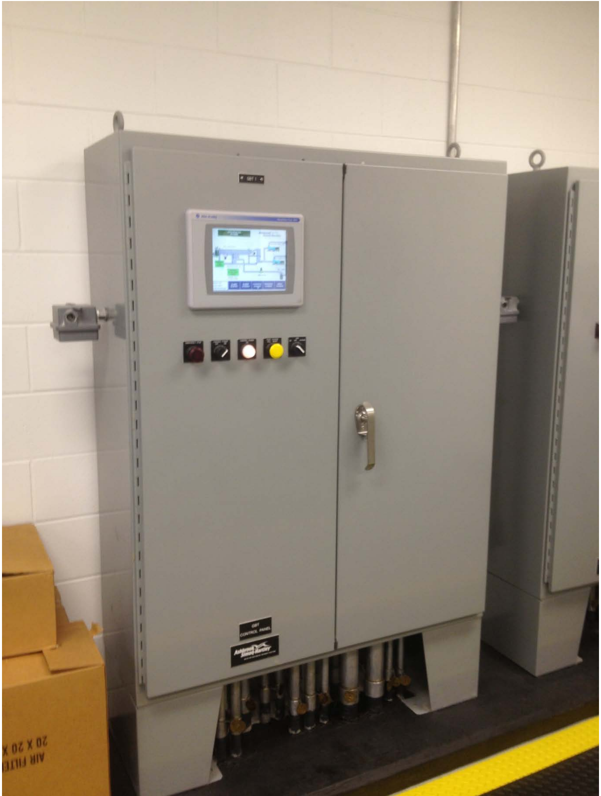
Exhibit No. 17 – Existing GBT Main Control Panel at the NEWRF
