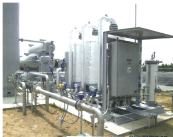
Figure 3-9. PSA and Vacuum Pump Skid and Buffer Vessels
