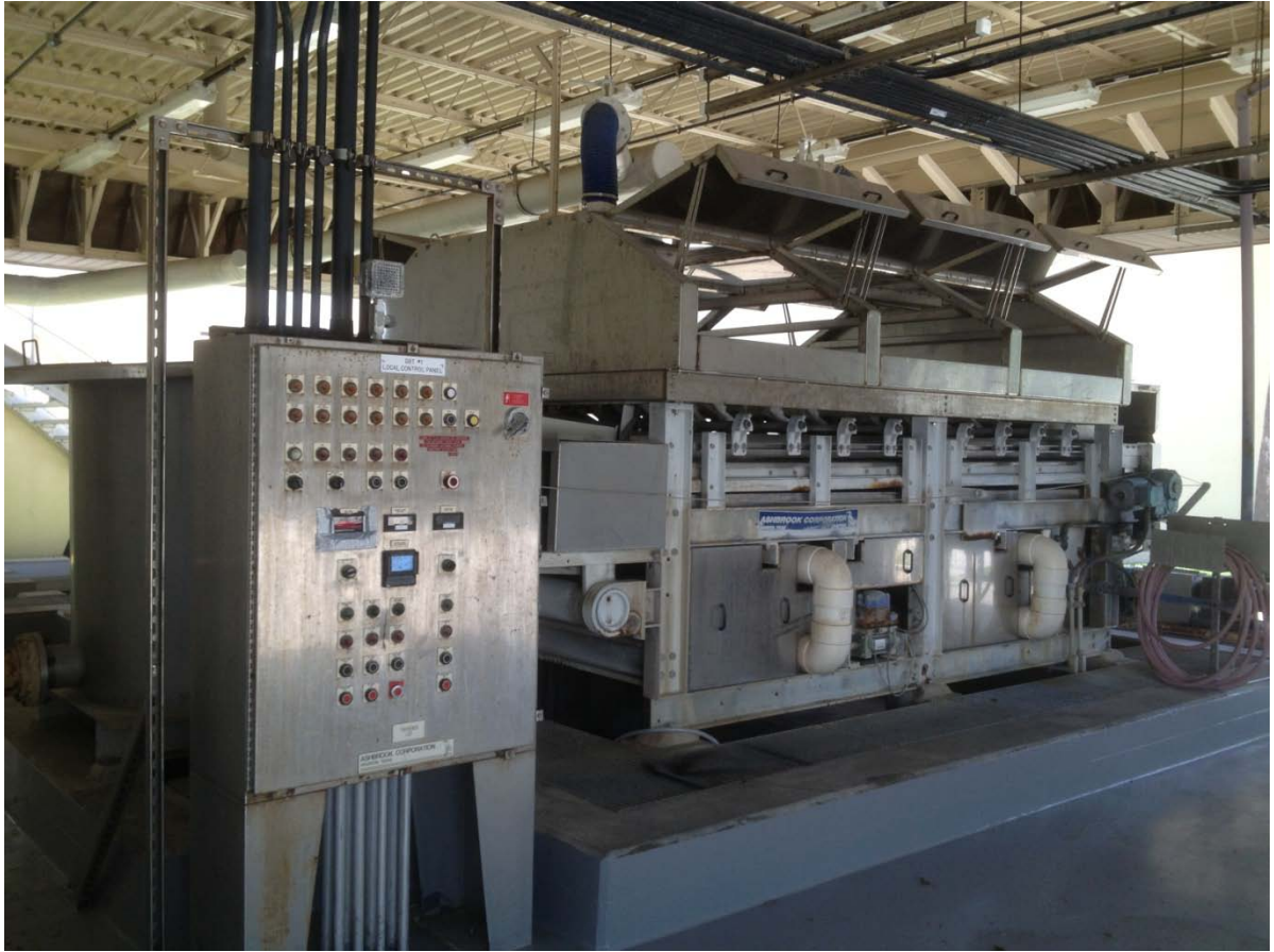
Exhibit No. 16 – Existing GBT Control Panel at the SWWRF
