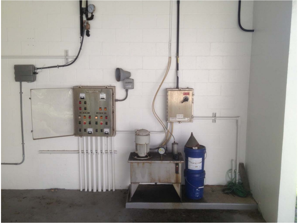
Exhibit No. 6 – Hydraulic Pack for the Existing GBT and GBT Feed Pump Control Panel at SWWRF
