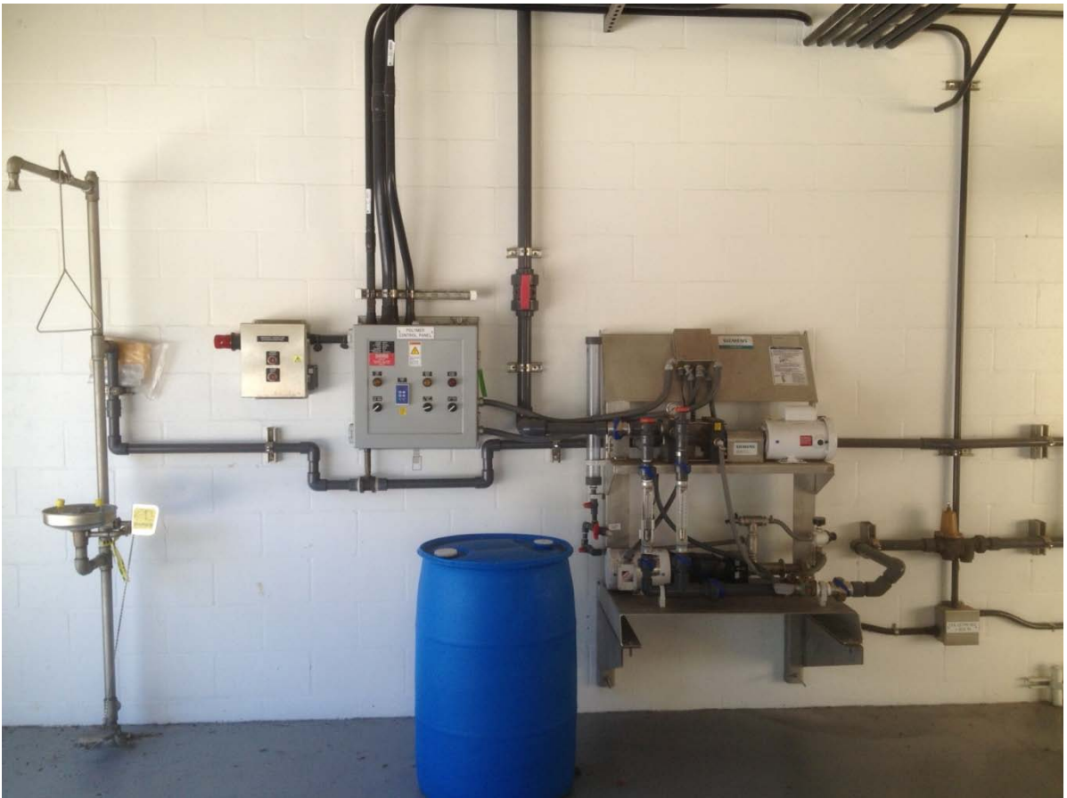
Exhibit No. 13 – Existing Emulsion Polymer Dilution and Feed System at the SWWRF
