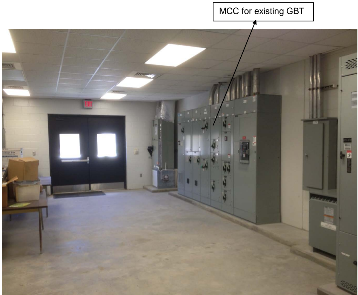
Exhibit No. 15 – Existing Electrical Building at the SWWRF
