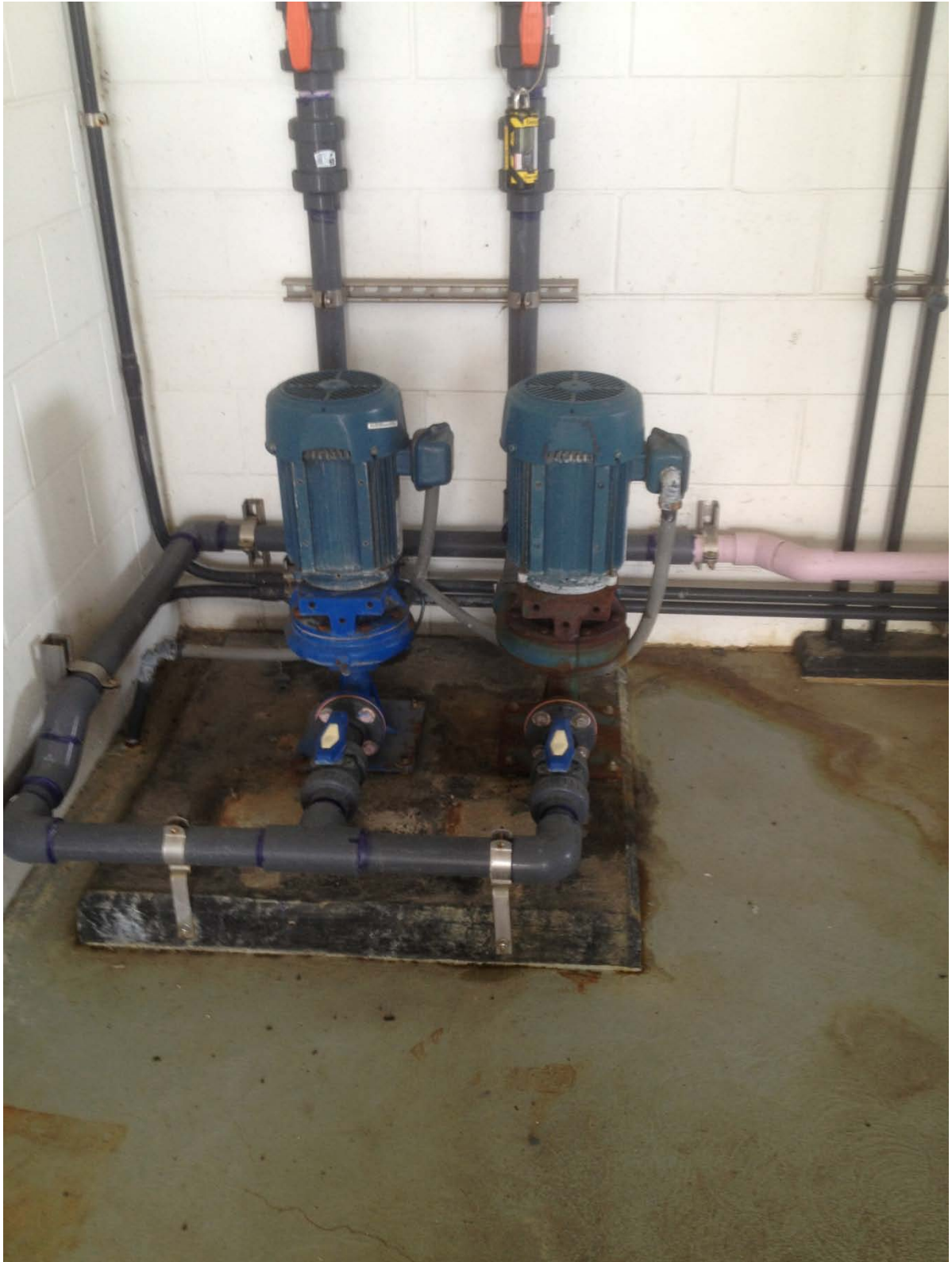
Exhibit No. 12 – Existing GBT Wash Water Pumps at the NEWRF
