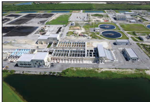
Clean Water State Revolving Fund provided loans for Miami-Dade South District Wastewater Treatment Plant.
