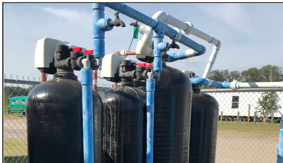
Filter Installation in Polk County
