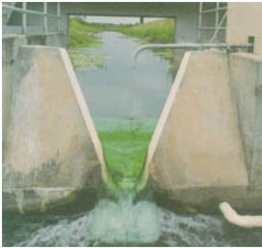
The H-flume outlet structure controls flows leaving the wetlands.
